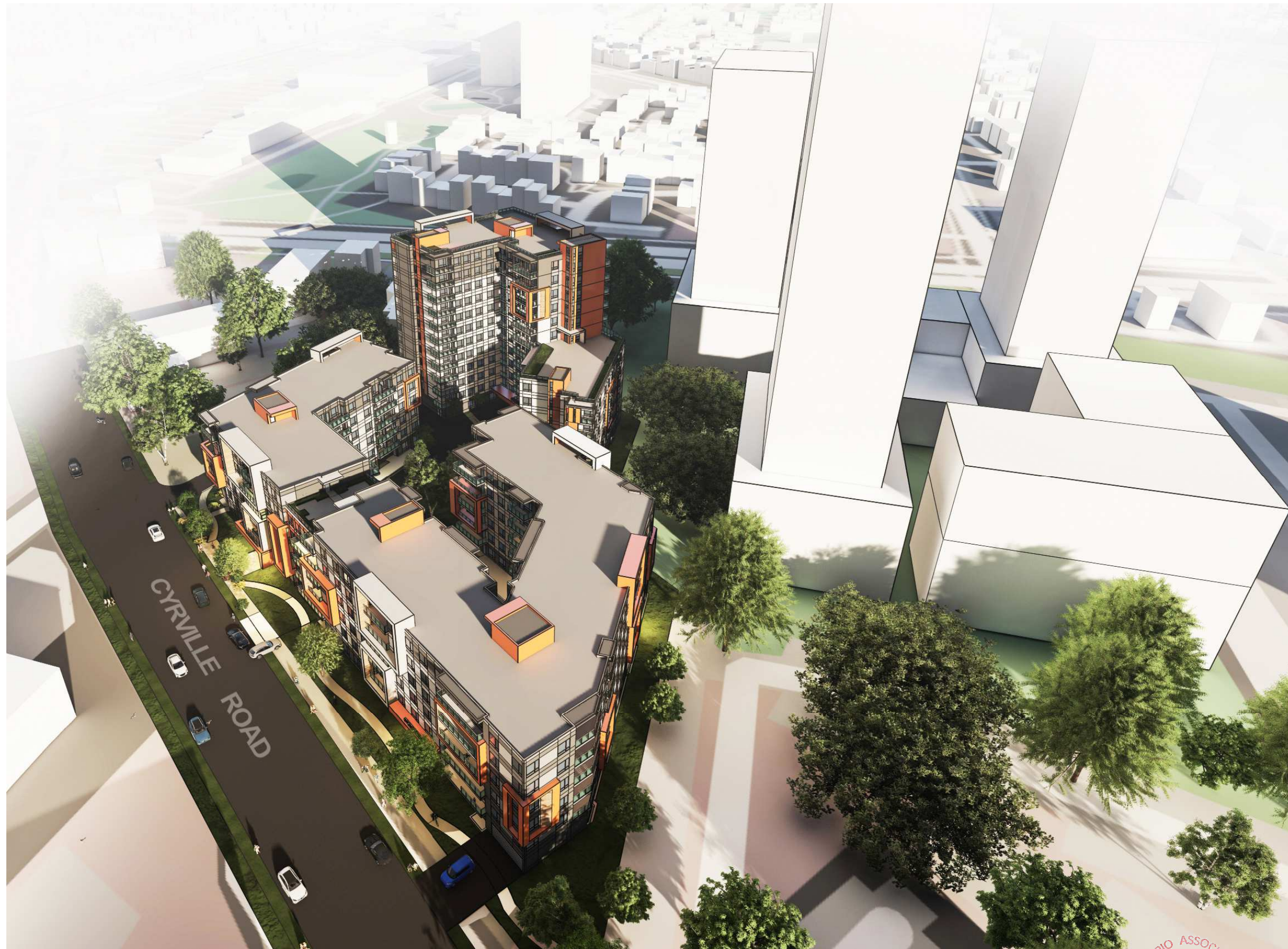
Aerial view – Looking Northwest
