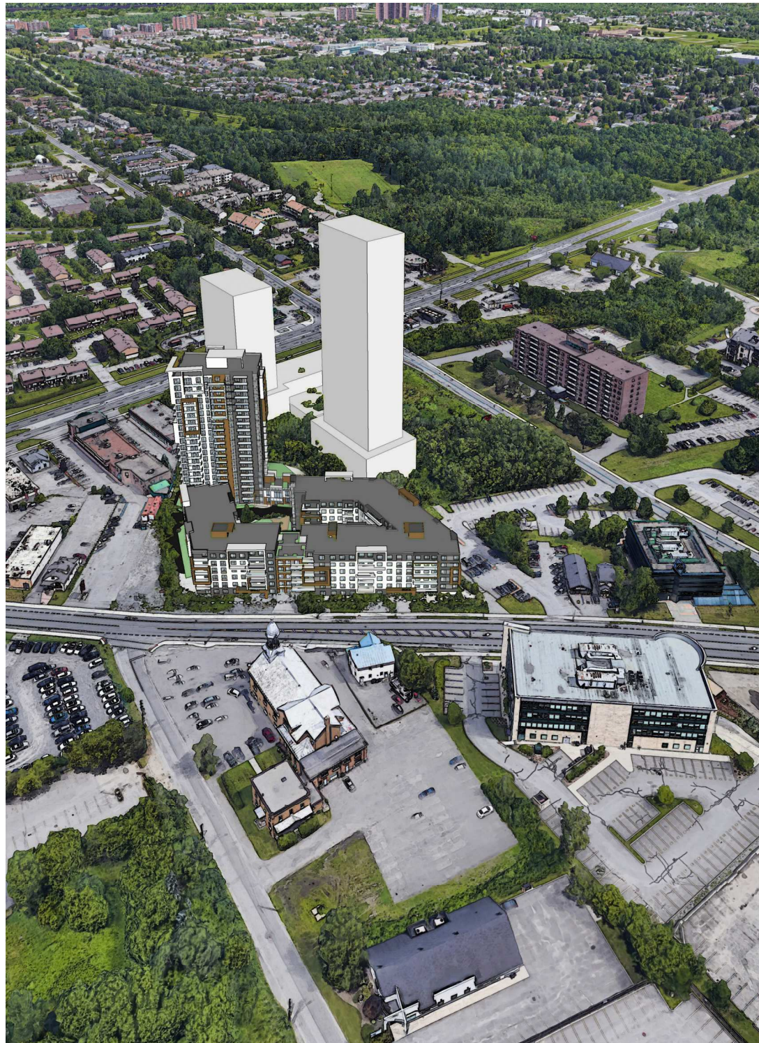
Aerial view – Looking Northeast
