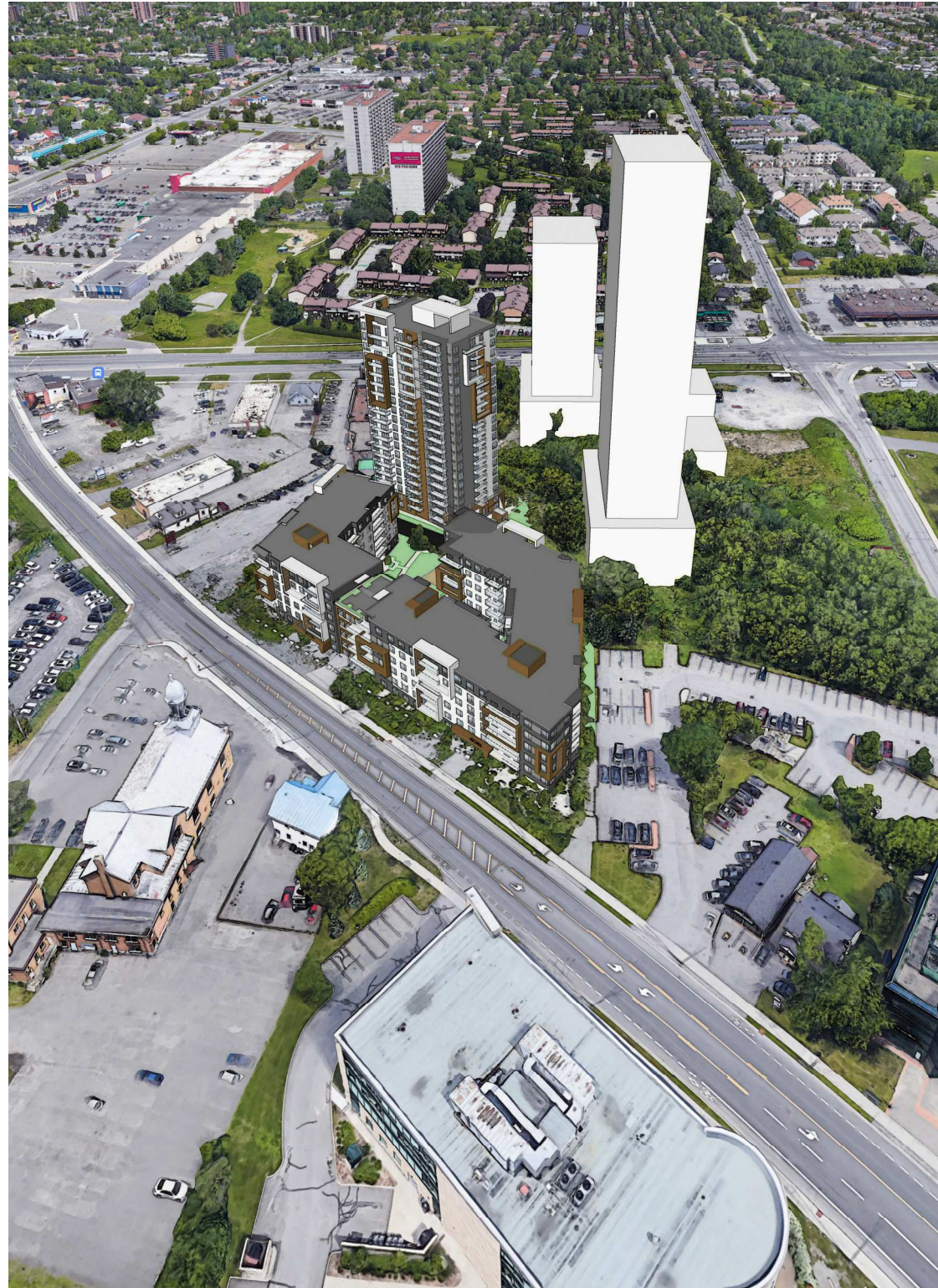
Aerial view – Looking Northwest
