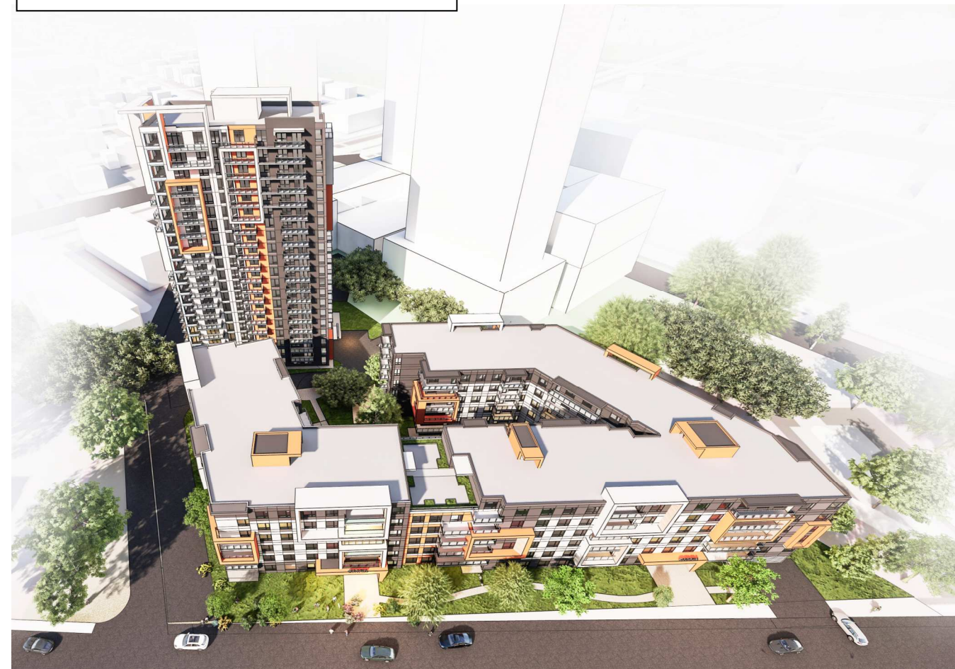
Aerial view – Looking Northwest
