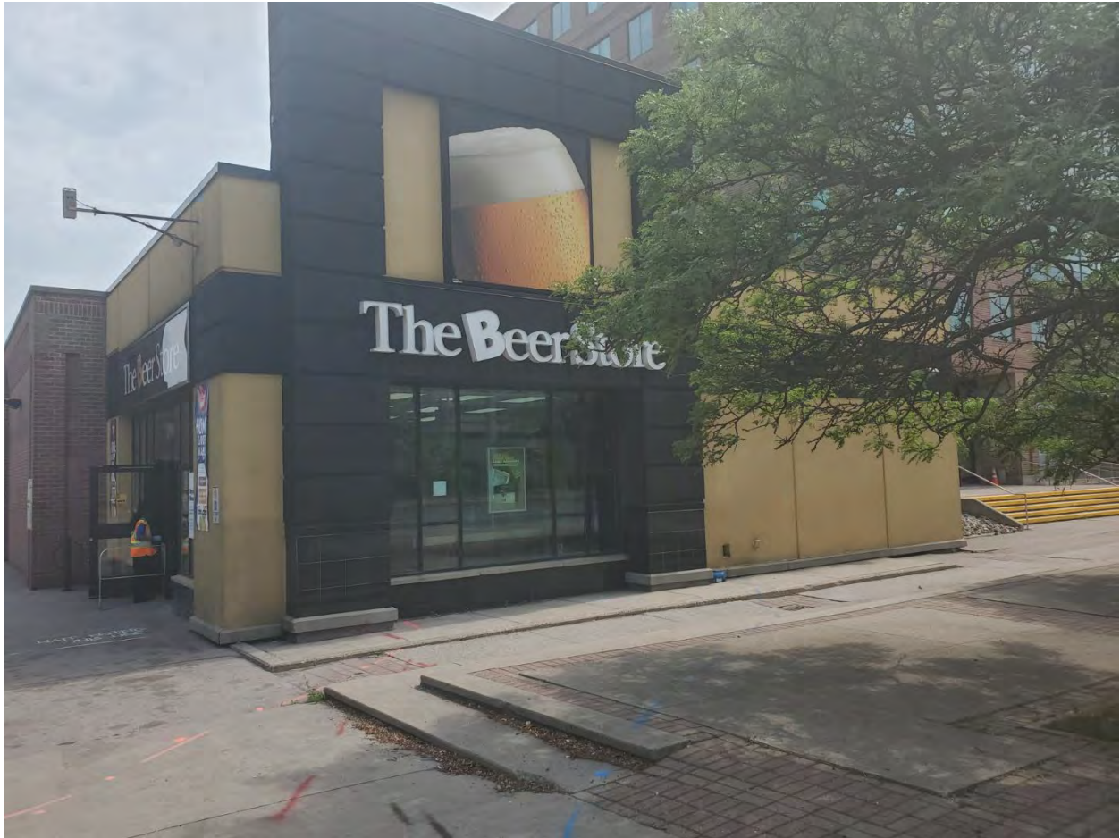
Photograph 1: Site north side.
