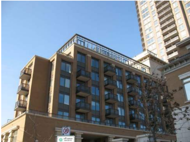
Sample Glass Parapets for Rooftop Terrace in Mississauga
