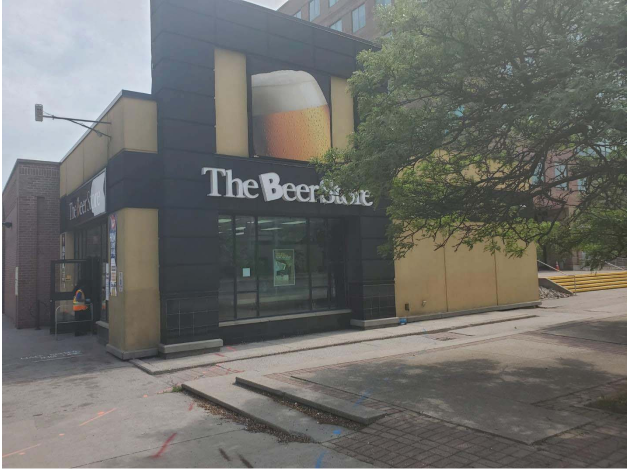
Photograph 1: Site north side.
