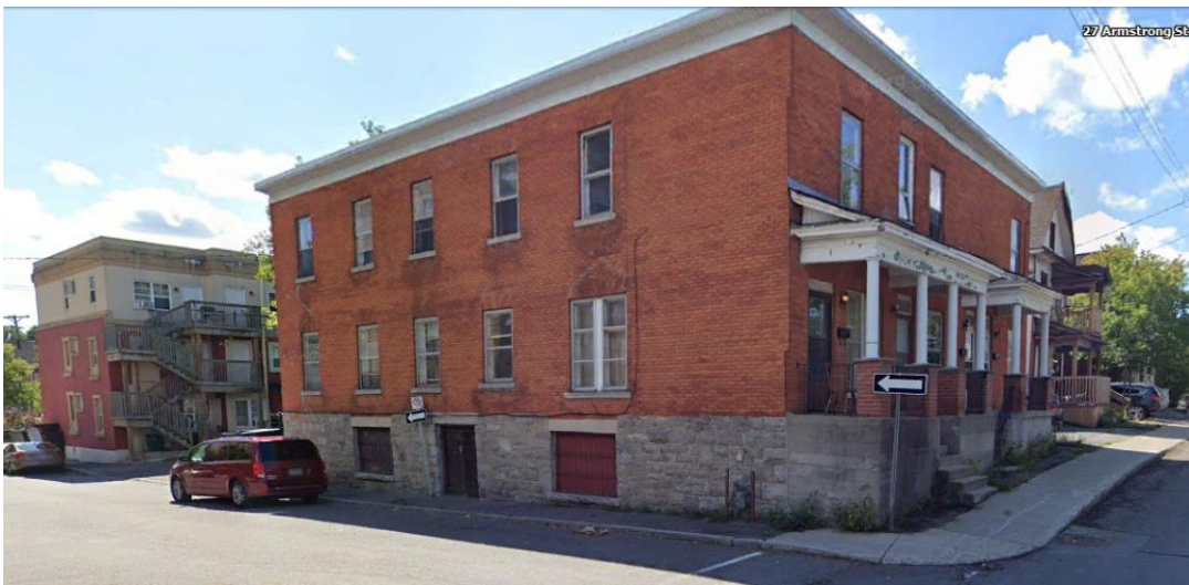
Figure 7: View of the row house at 26 Armstrong (right) and 967 Wellington (left) with no accessible frontage on Hilda Street. The building is typical of the area’s character– two and three storey brick clad building, masonry foundation with flat roofs set on the property line. Both buildings on this block of Hilda Street are slated for demolition. Source: Google
