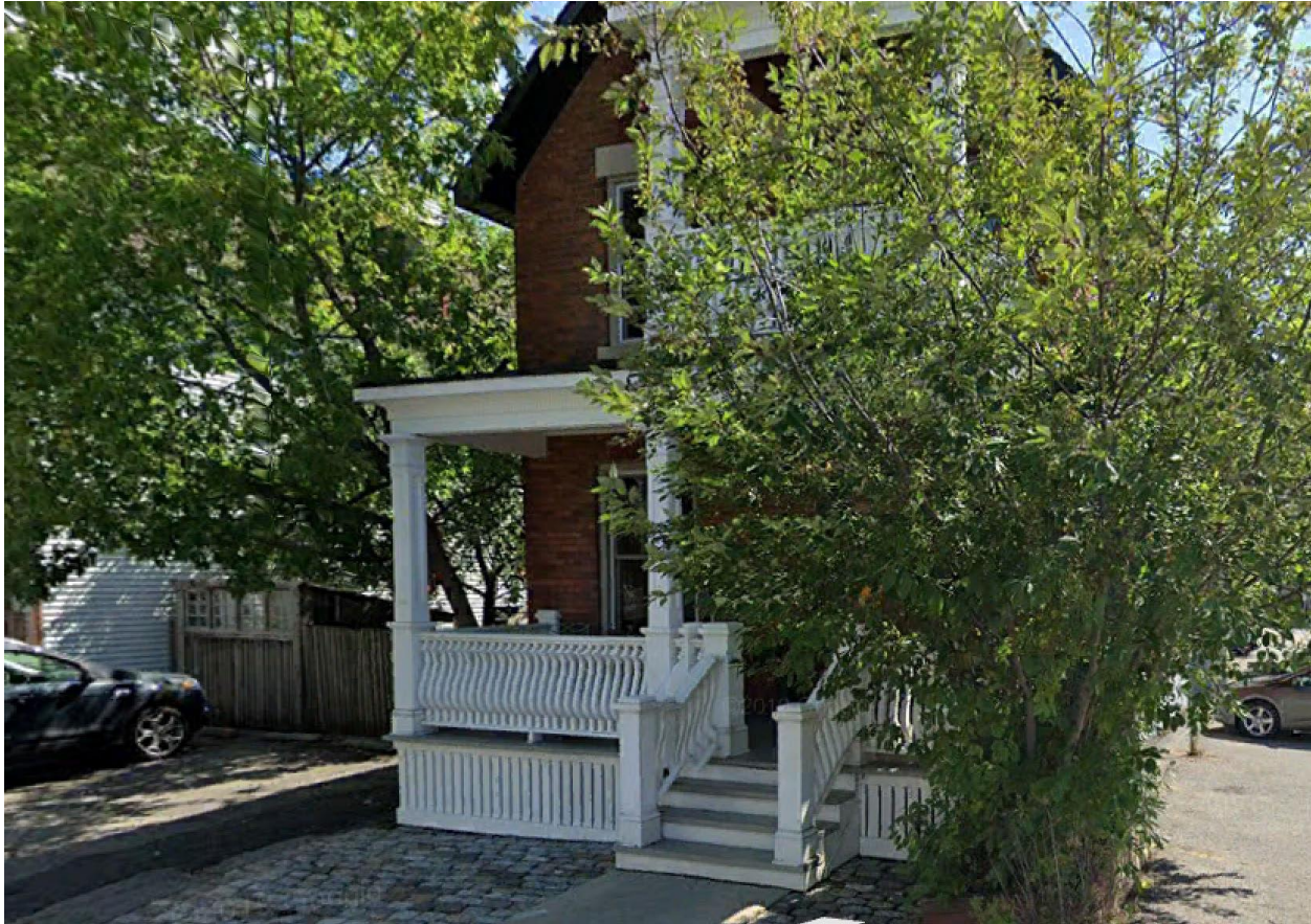
Figure 14: Street view of 40 Armstrong Street. Note the handsome wood porch with a second-floor covered balcony Source: Google Earth
