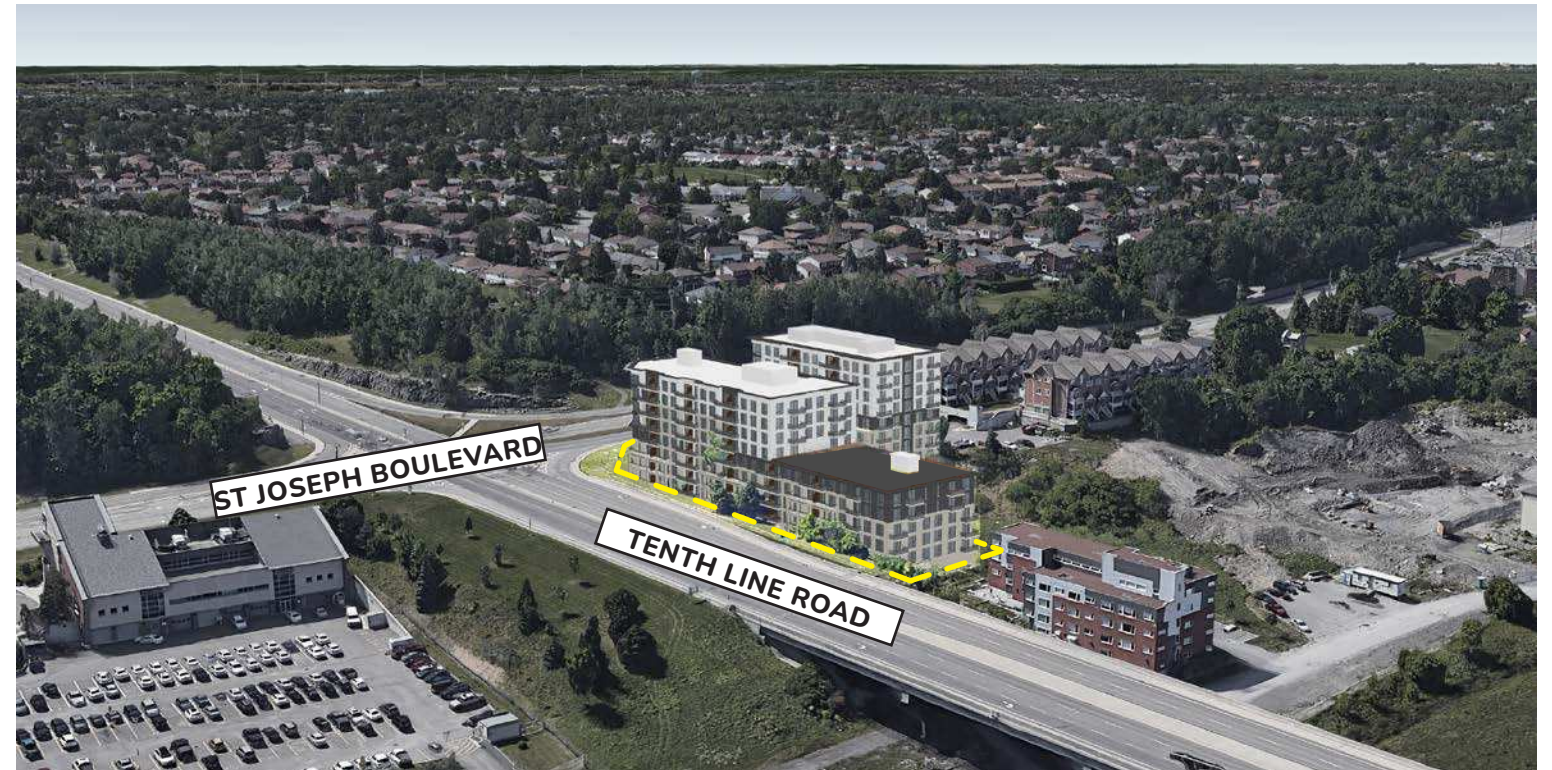
2 - SOUTHERN AERIAL VIEW FROM TENTH LINE ROAD
