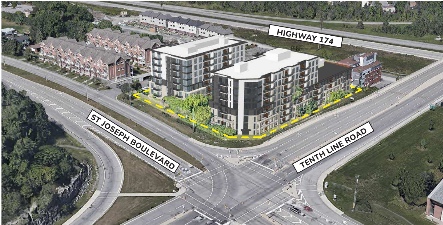
1 - AERIAL VIEW FROM INTERSECTION OF ST JOSEPH BOUL. & TENTH LINE RD
