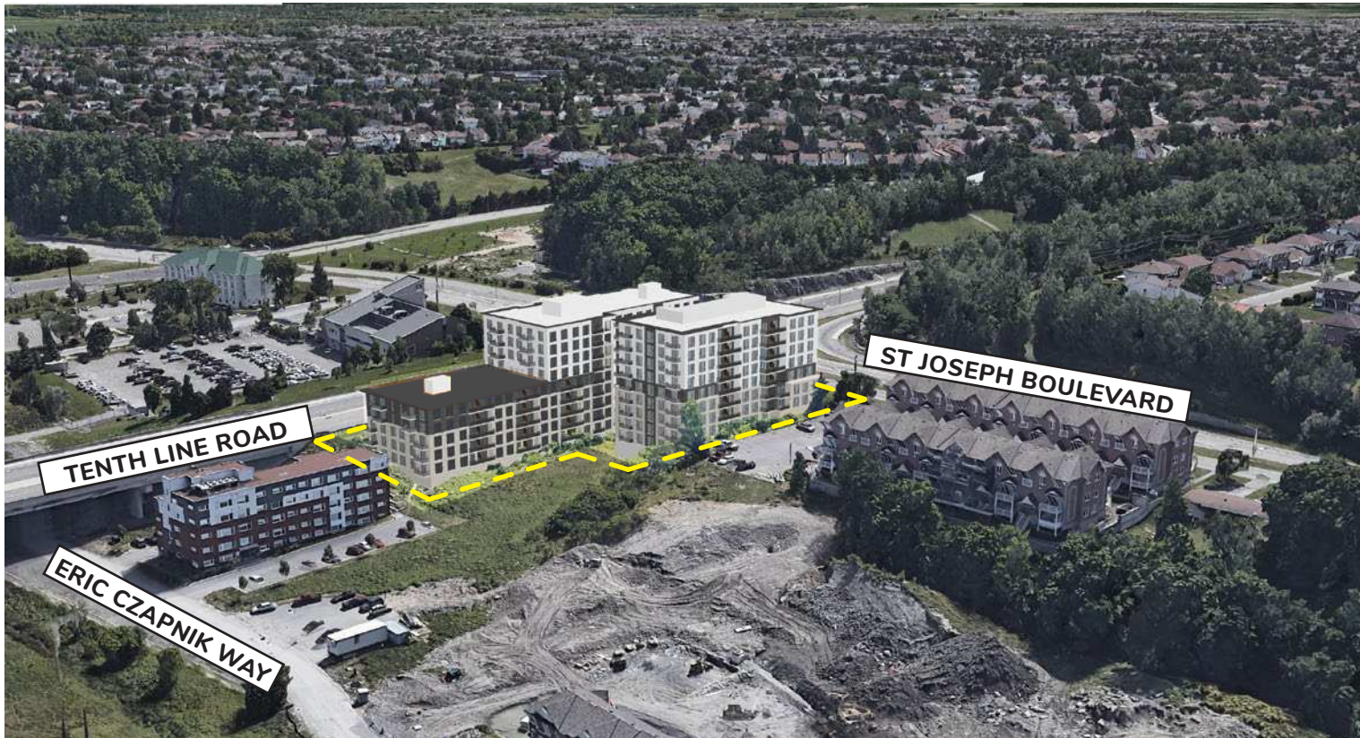
3 - AERIAL VIEW FROM NORTHERN END OF SITE ABOVE ERIC CZAPNIK WAY
