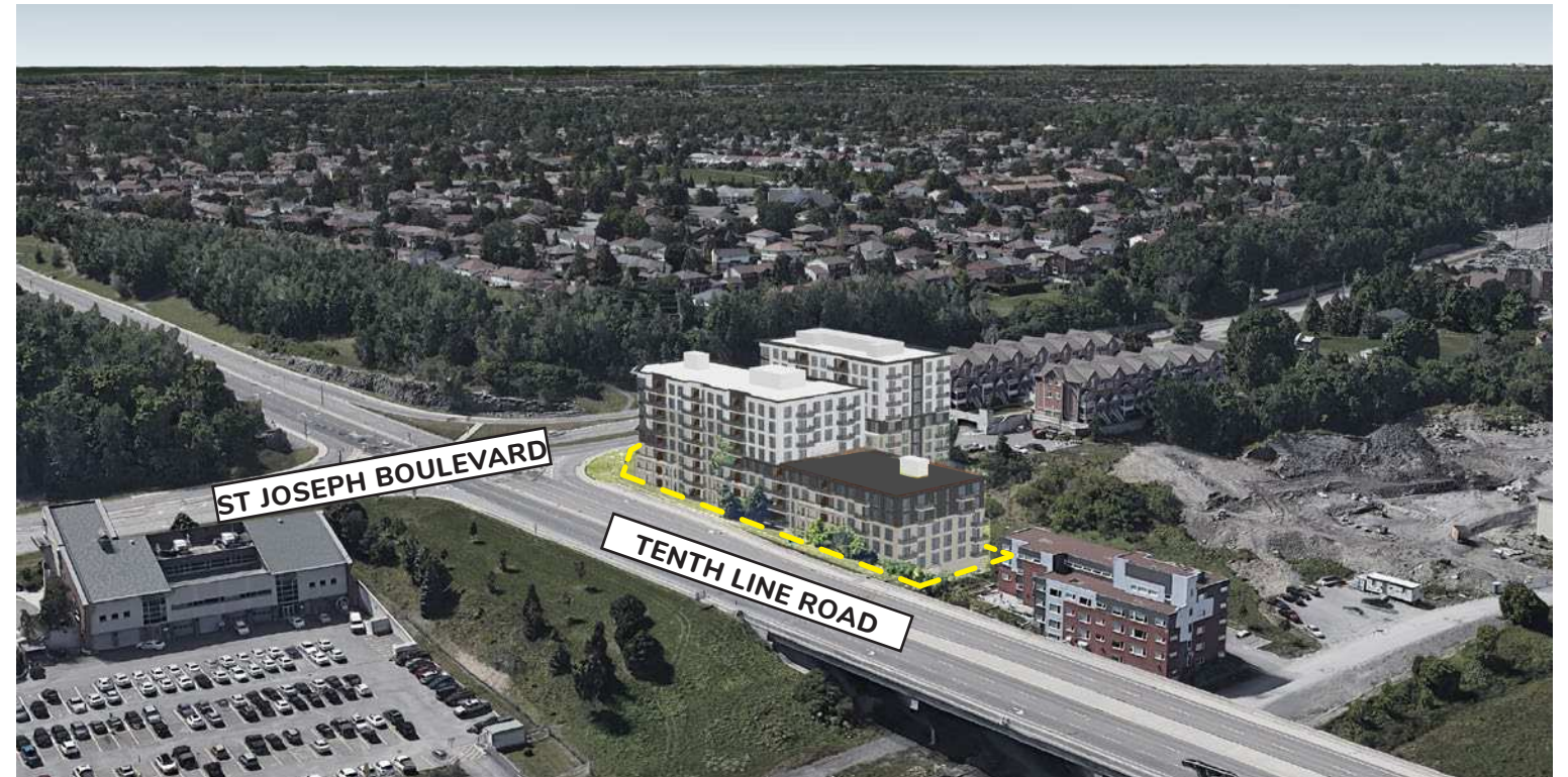
2 - SOUTHERN AERIAL VIEW FROM TENTH LINE ROAD
