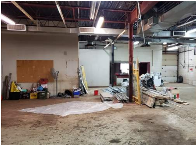
Photo 9: View of the northern portion of the Site building, facing away from Coldwater Road. Photograph taken facing north.
