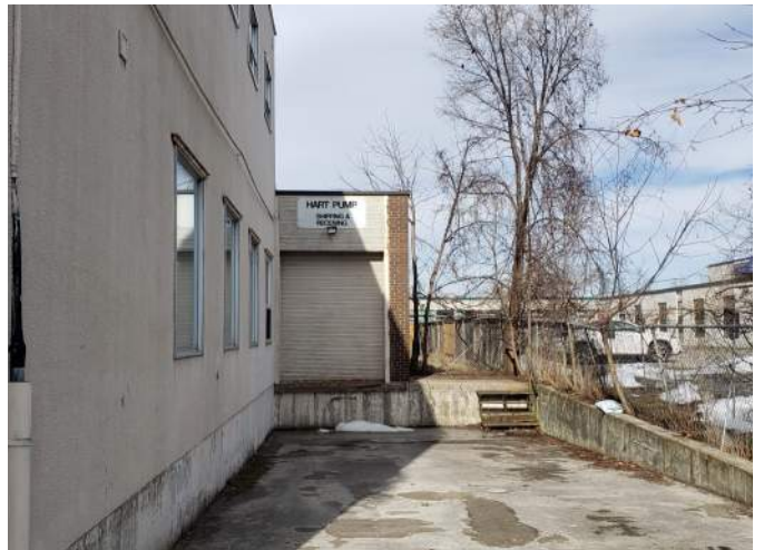
Photo 4: View of the eastern property line and former shipping dock. Photograph taken from Coldwater Road facing north.
