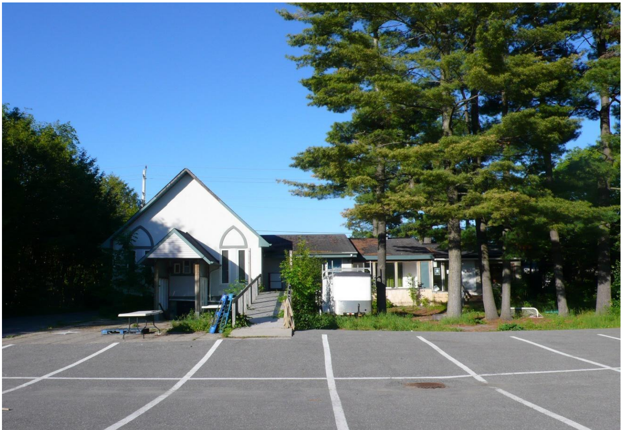
Rear of existing building at 572 Moodie Drive (June, 2019)
