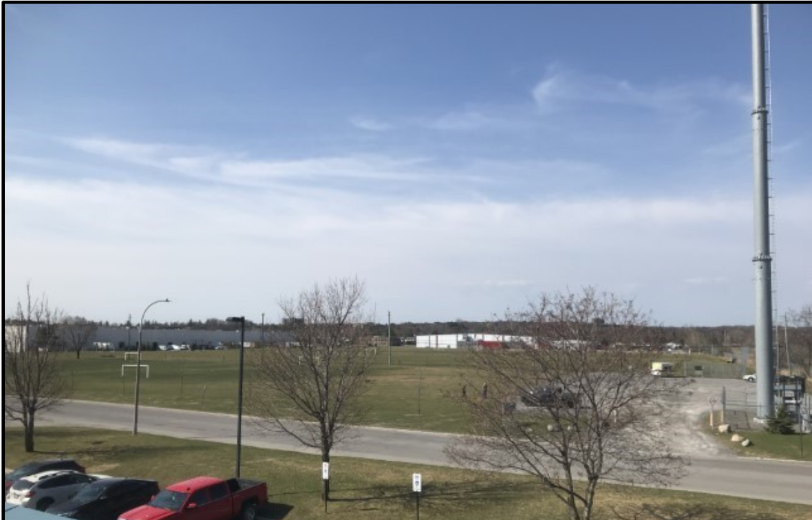
Photo 5: West-facing view of the communications tower and park.
