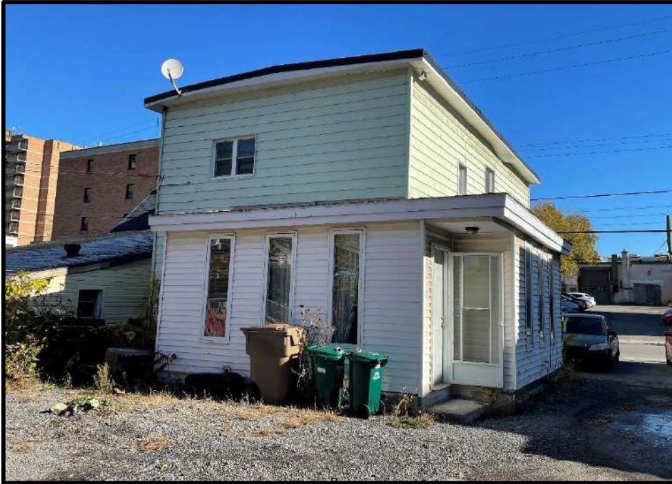
Photograph 3: View of southwestern side of the residential dwelling, facing northeast from the gravel parking area.
