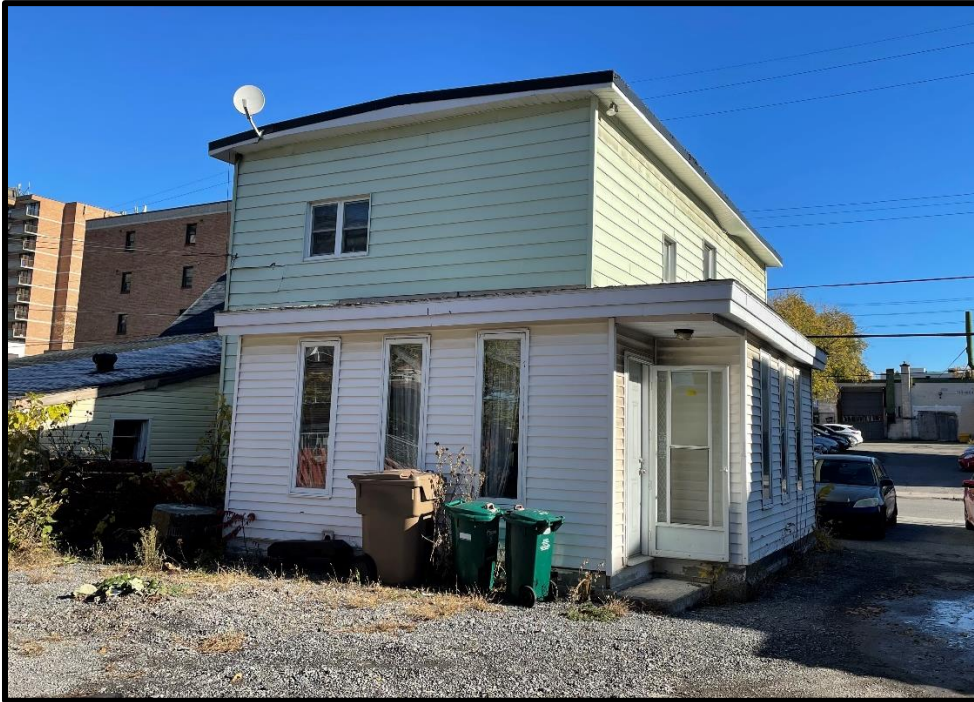
Photograph 3: View of southwestern side of the residential dwelling, facing northeast from the gravel parking area.
