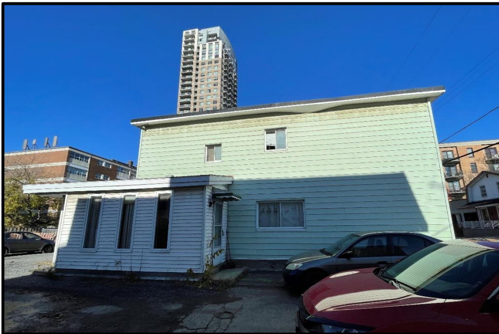
Photograph 2: View of the southern side of the residential dwelling, facing north from the asphalt parking area.
