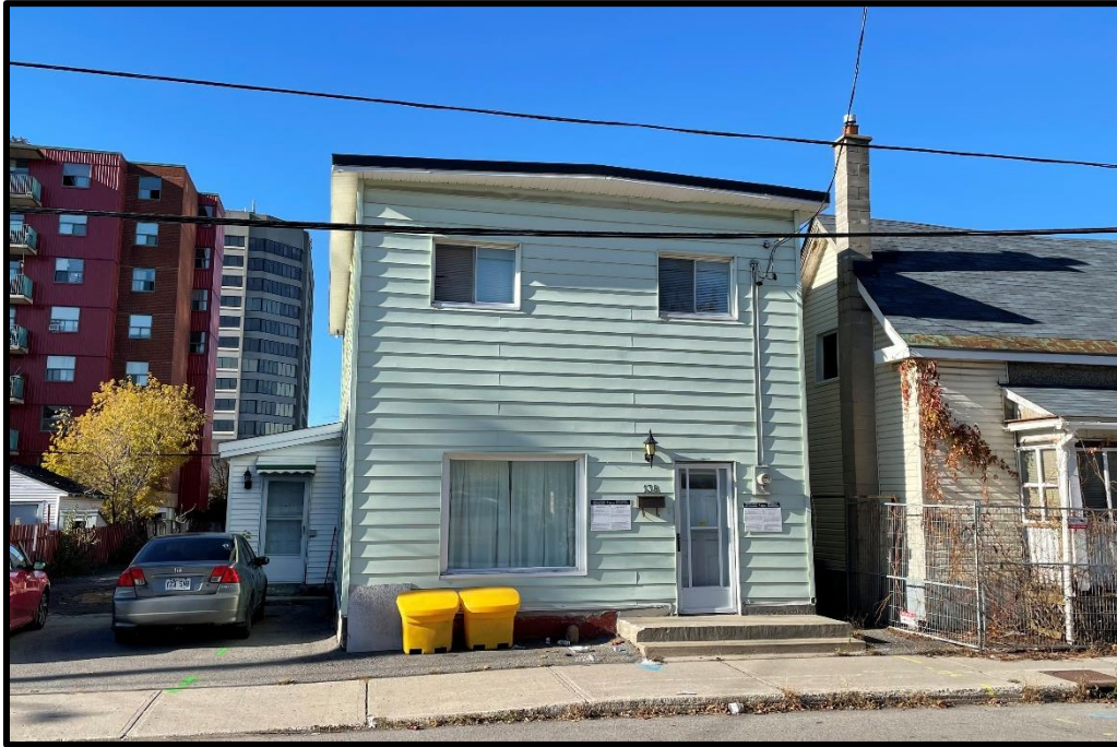
Photograph 1: View of the eastern side of the residential dwelling, facing west from Forward Avenue.
