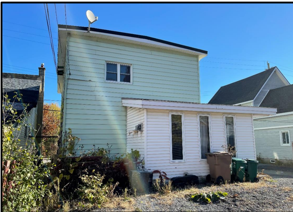
Photograph 4: View of western side of the residential dwelling, facing east from the gravel parking area.
