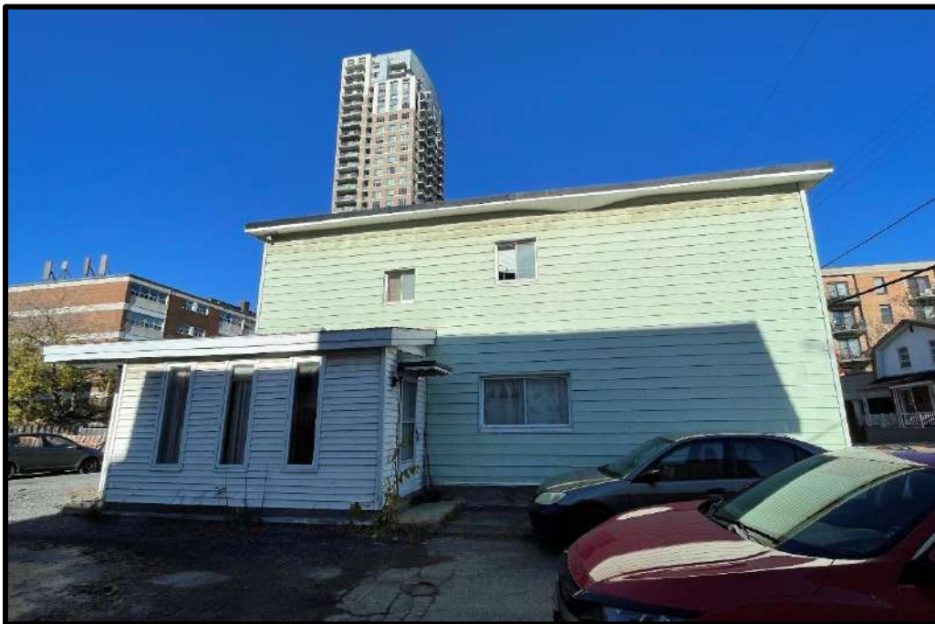
Photograph 2: View of the southern side of the residential dwelling, facing north from the asphalt parking area.
