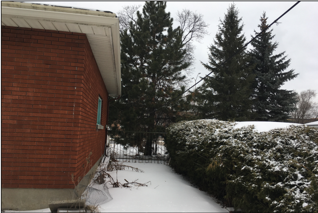
Photo 5: East side of on-site residence, looking northwest from rear.
