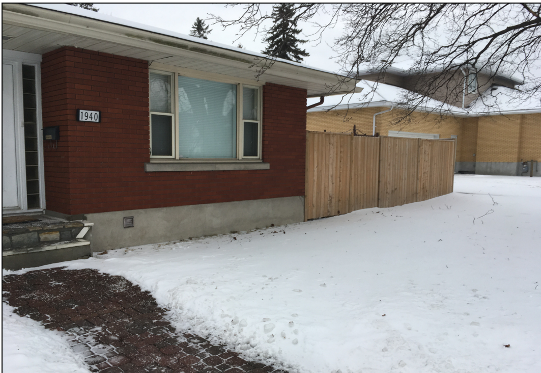
Photo 2: View of on-site and adjacent residences, looking south.
