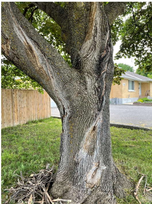
Figure 2: Close up of spiral cracking on tree 1
