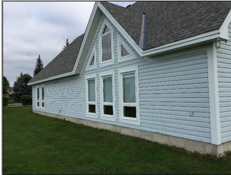
Photo 1 – Site Building A (south elevation).
