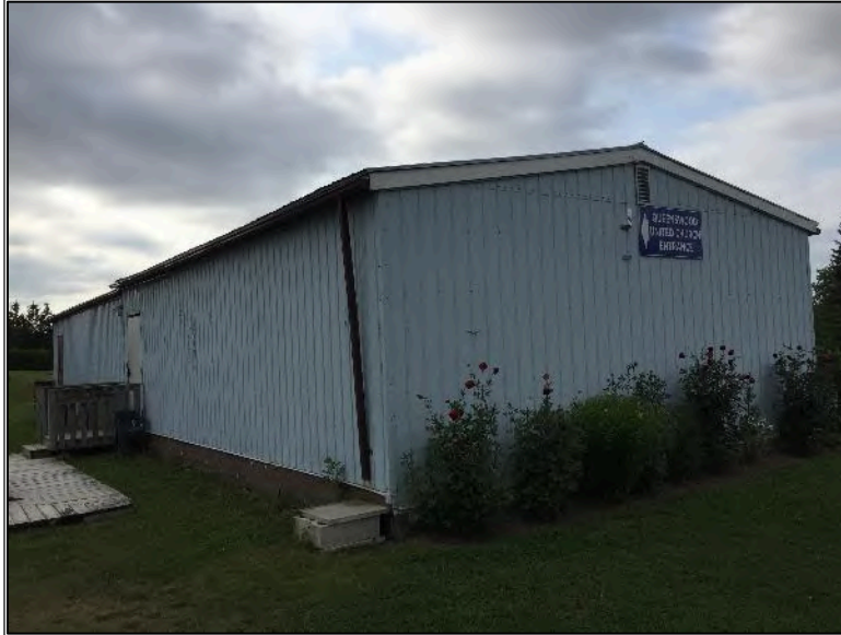
Photo 3 – Site Building B (north and west elevations).
