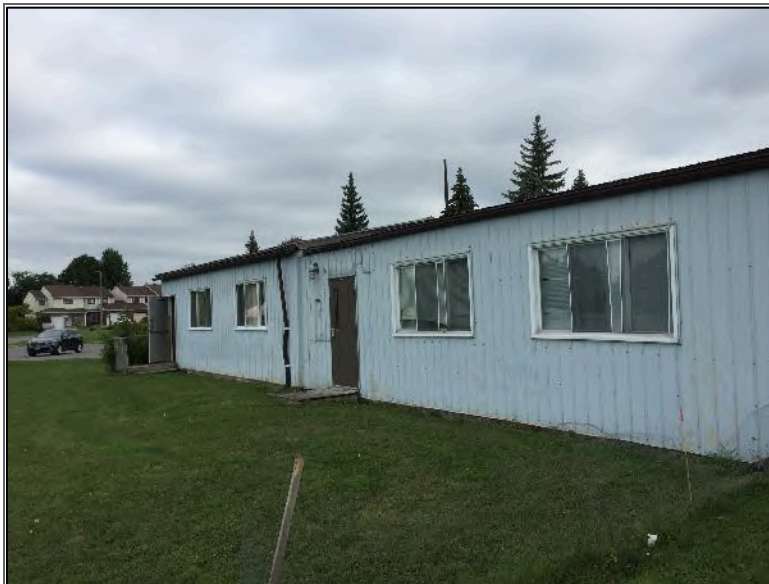
Photo 4 – Site Building B (south elevation).
