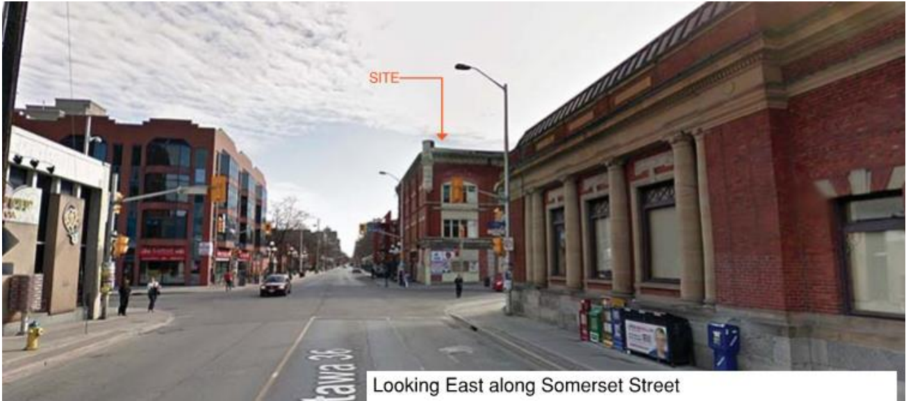
FIGURE 8. STREETVIEW OF THE SITE FACING NORTHEAST (GOOGLE STREETVIEW)
