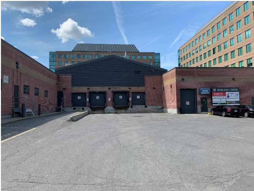
Photo 3: Loading Dock (North of the Phase One Property) - Facing West
