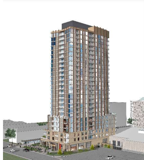
View Looking Southwest
