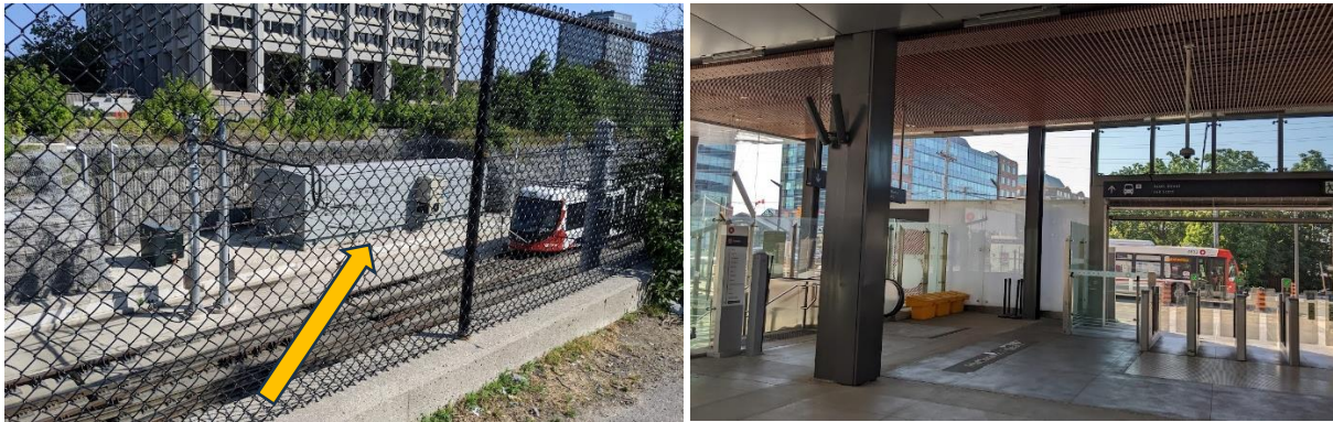
Photo 5: Left: View of TPSS (arrow added), facing northeast. Right: LRT access to street level (Scott St.), facing southeast.
