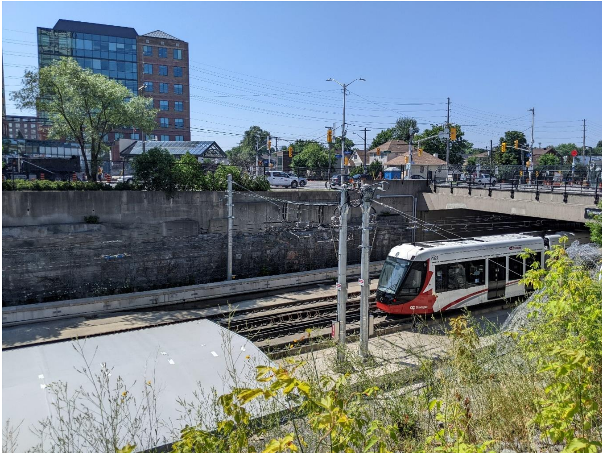
Photo 4: View of LRT trench and Holland Avenue bridge, facing southwest towards Scott Street and Holland Cross.
