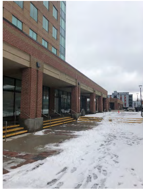
Photo 2 – Southern side of the Site and adjoining structures, looking northeast
