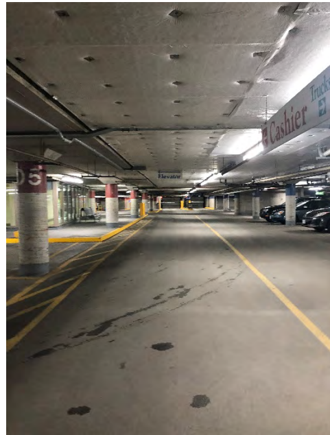
Photo 16 – First sub-level parking, facing east, looking at eastern entrance
