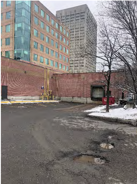
Photo 7 – Loading bay area north of the Site, looking northwest
