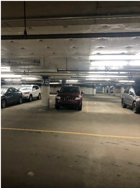
Photo 15 – First sub-level parking
