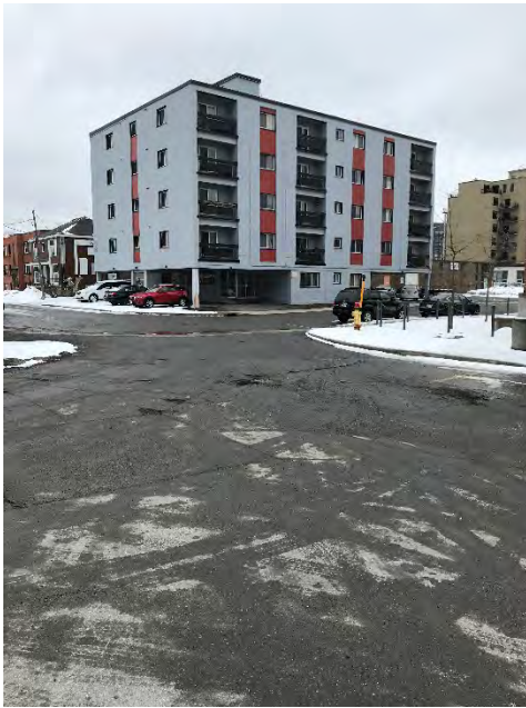
Photo 1 – Apartment building (1 Hamilton Avenue North), east of the Site, looking southeast
