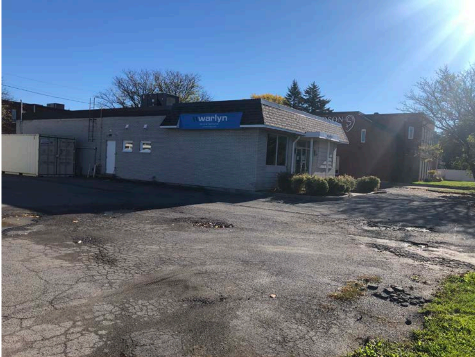
View from site facing south of commercial office building located south of site.
