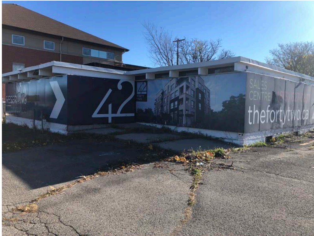
View of building converted into a sales center
