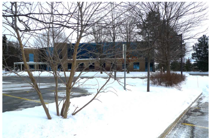
Adjacent existing commercial development
