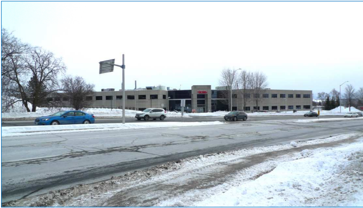
View across Palladium Drive
