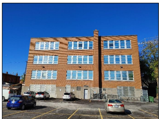
Figure 2-3 Site, looking north
