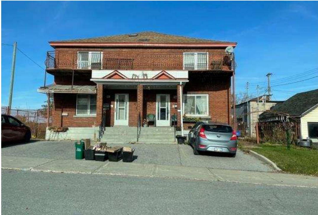
Photograph 1: View of the 15 and 17 Larch Street, looking north.
