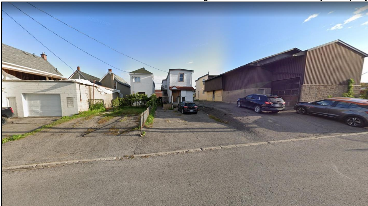
Figure 4. Land uses south of Subject Property
