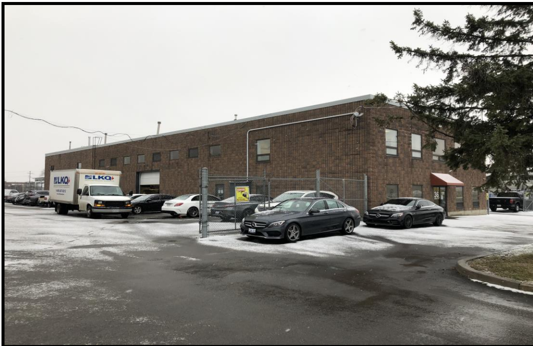
Photograph 4: View of the eastern portion of 36 Jamie Avenue, facing south.
