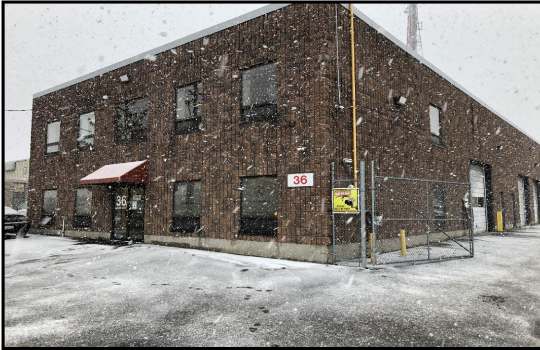
Photograph 3: View of the northern portion of 36 Jamie Avenue, facing south.
