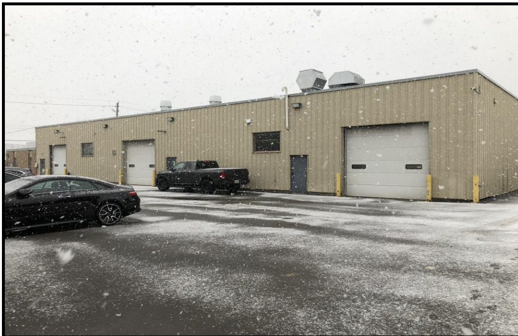
Photograph 2: View of the western portion of 40 Jamie Avenue, facing east.
