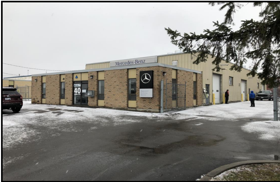
Photograph 1: View of the northern portion of 40 Jamie Avenue, facing south.
