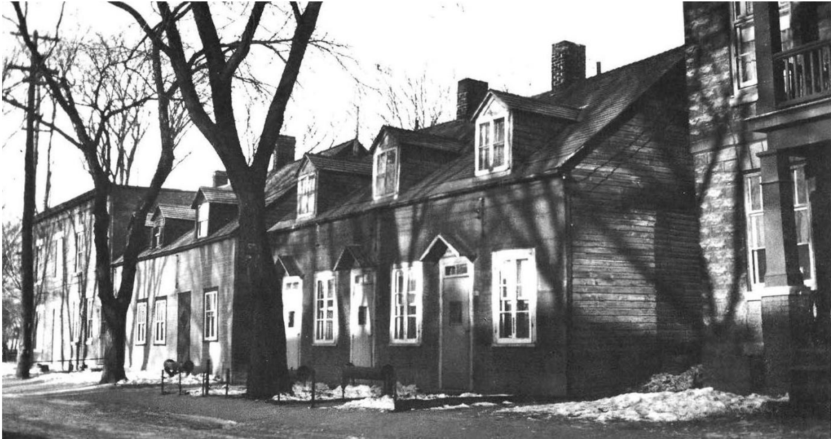
Figure 15: Historic photograph (n.d.) of workers cottages in Lowertown. Note the exterior finishes – wood siding and shingles, baseboard at the base of the wall and simple corner board and window and door trim. Note the entrance canopies, the minimal eave overhang, and the single hung multi-pane sash. Source: Newton, M. (1980). The Search for Heritage in Ottawa's Lower Town . Urban History Review / Revue d'Histoire Urbaine , 9 (2), 21–37. https://doi.org/10.7202/1019334ar
