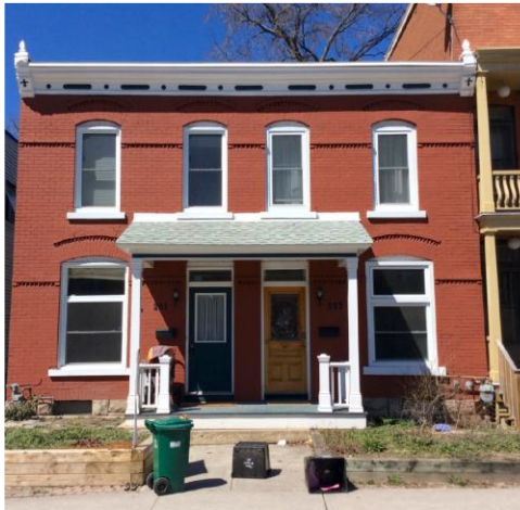
Figure 27: Elevation of 281-283 Clarence illustrating many of the same features. Built in 1898 in an Italianate style including two storey, flat roof, double entrance doors, corbelled brick banding, arched headed windows scaled between ground and second floor, masonry foundation, painted red brick and heavy metal cornice. Source City of Ottawa inventory.
