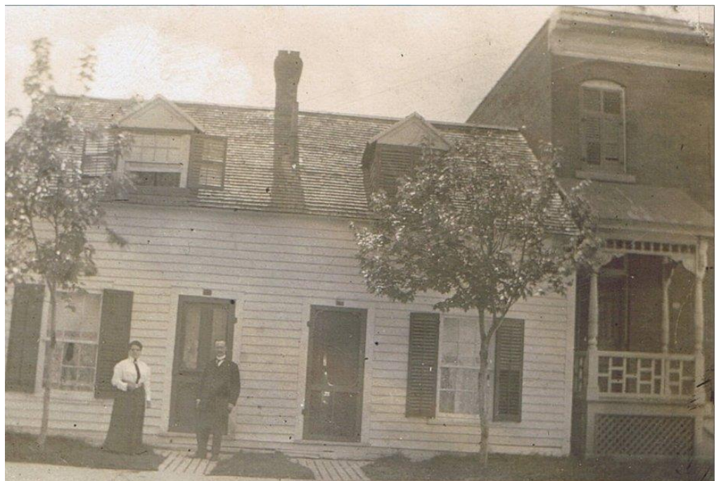
Figure 14: Historic photograph (n.d.) of a worker's cottage and a brick clad house in Lowertown. Note the exterior finishes – wood siding and shingles, baseboard at the base of the wall and simple corner board and window and door trim. Note the lack of entrance canopies, the minimal eave overhang, and the single hung multi-pane sash. Note the cornice detailing on the brick building. Source: Library and Archives Canada.
