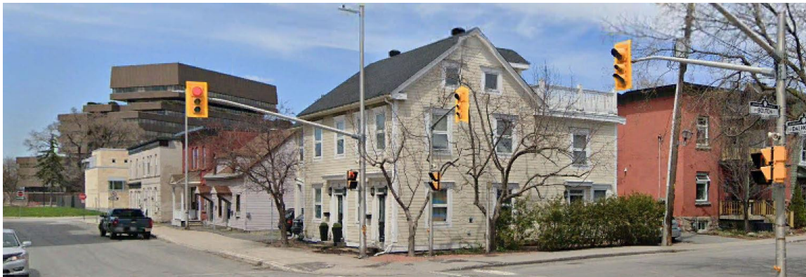
Figure 6: View looking north on Dalhousie Street at the corner of Bolton Street to the mid-block development site (below the traffic light). Source: Google Earth
