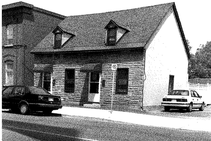
Figure 26: view of the 113-115 front façade from the 1992 inventory form illustrating the rendered stucco on the south elevation and the angel stone treatment on the front façade. City of Ottawa inventory form.
