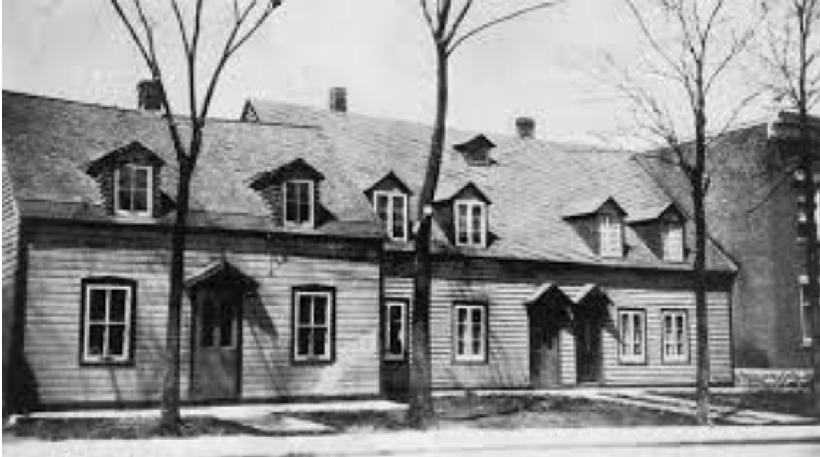
Figure 17: Historic photograph of worker's cottages in Lowertown. n.d. The finishes and detailing – wood-siding, roof finishes dormers, windows both doubles hung (left) and casement (right) and simple entrance canopies are typical of the area. Source: Canadian Inventory of Historic Buildings (CIHB)
