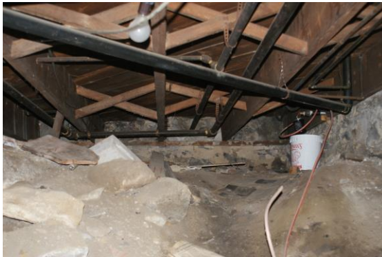
Figure 26: View documenting the crawl space below the worker's cottage. Source: Commonwealth
