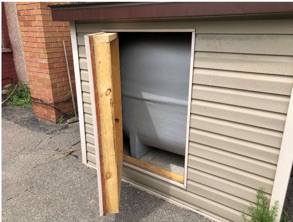
Photograph 4: Out-of-service fibreglass AST at rear of 111 Dalhousie Street.
