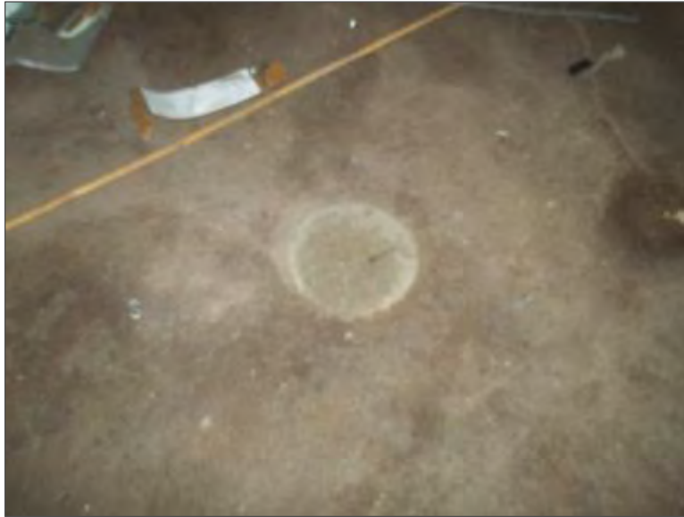
Photo 9 – Evidence of a former borehole within the Site Building.
