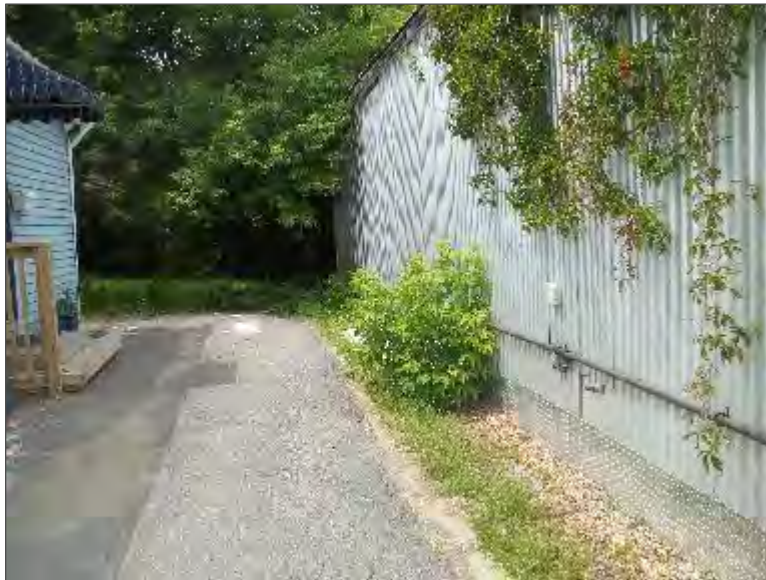
Photo 4 – Site Building (southeast elevation).
