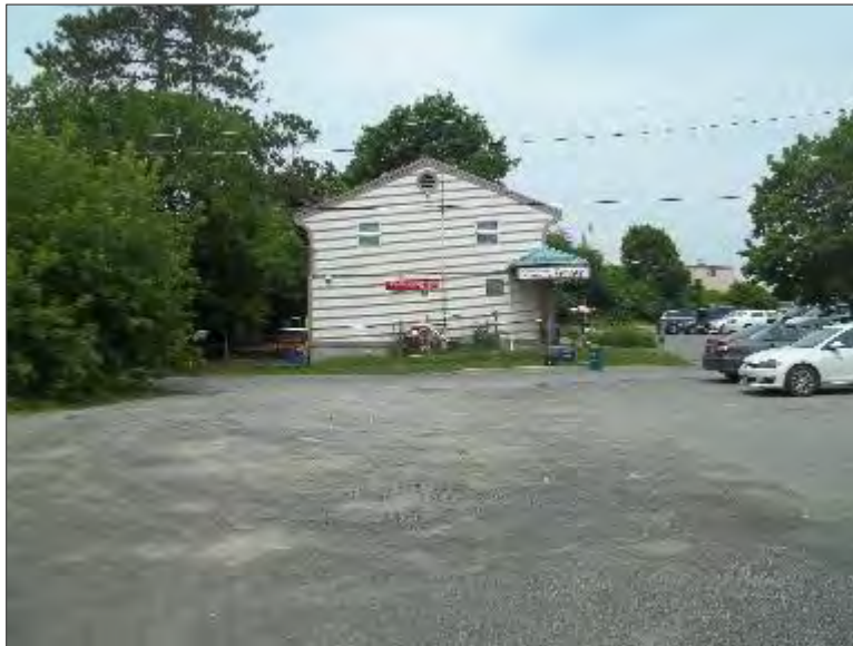
Photo 2 – Site Building (southwest elevation) and south/southwest portion of the Site.
