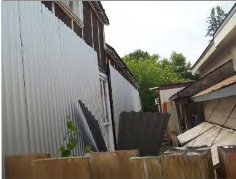
Photo 1 – Site Building (northwest elevation).
