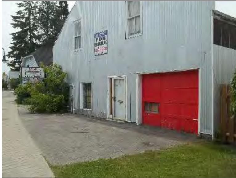
Photo 3 – Site Building (northeast elevation).
