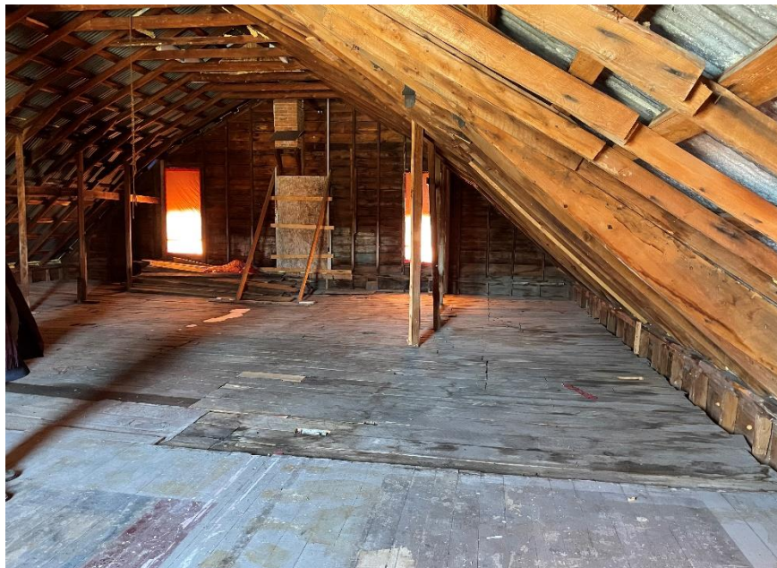
Photo 4 – Second level, facing west.
