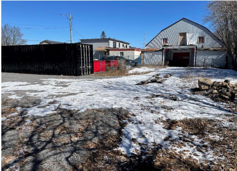
Photo 1 – Yard and west elevation of Site Building.
