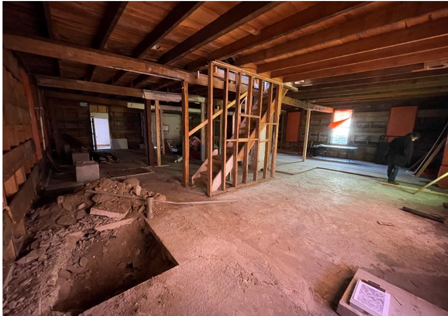
Photo 3 – Main level interior, facing west.
