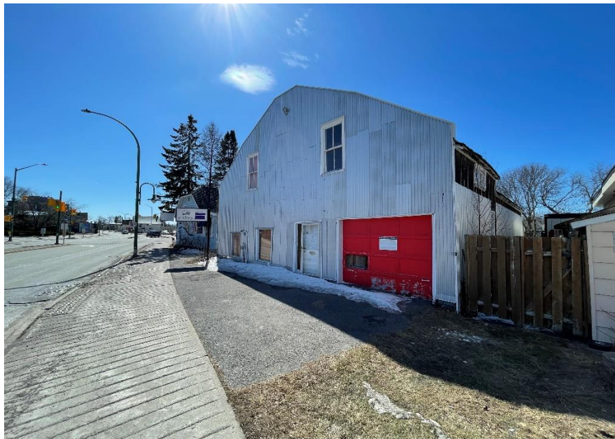
Photo 2 – East and north elevations.
