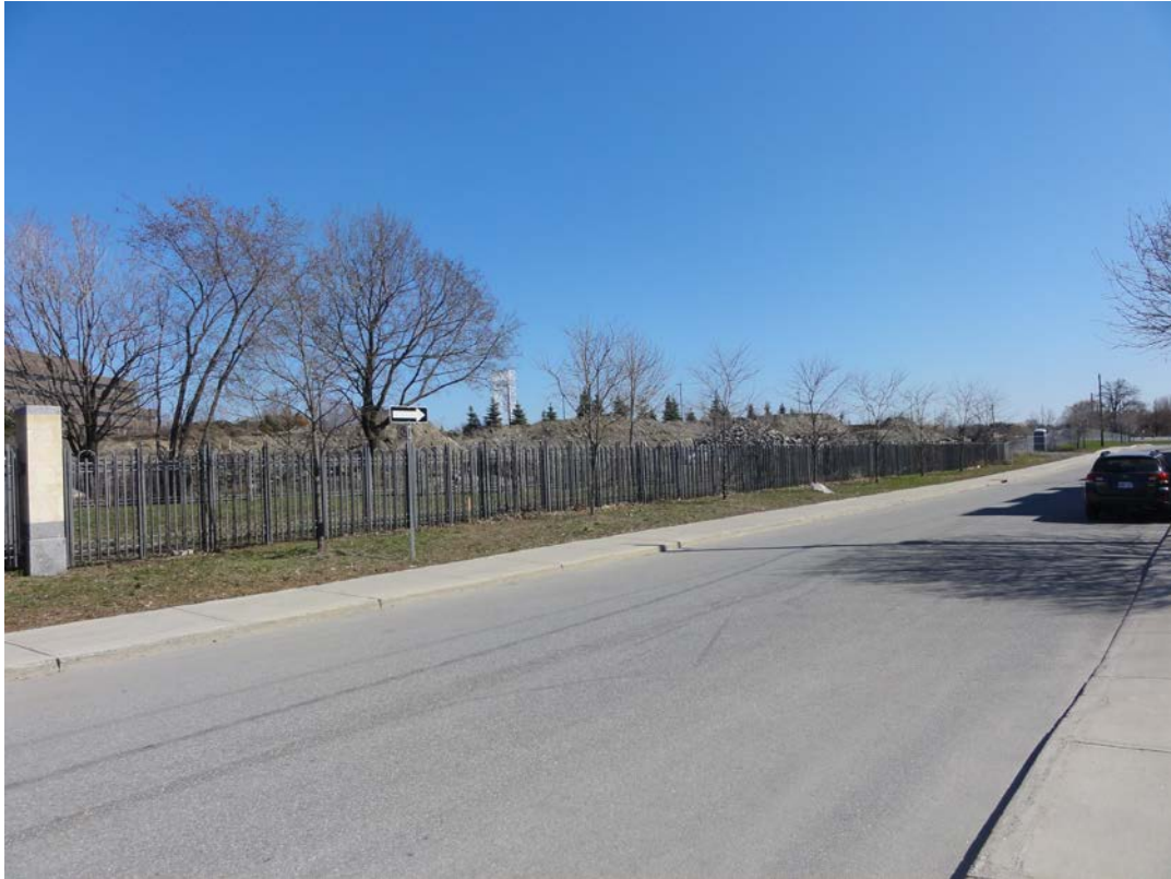
Photo 3: Looking northeast along the southern property line (April 22, 2013).
