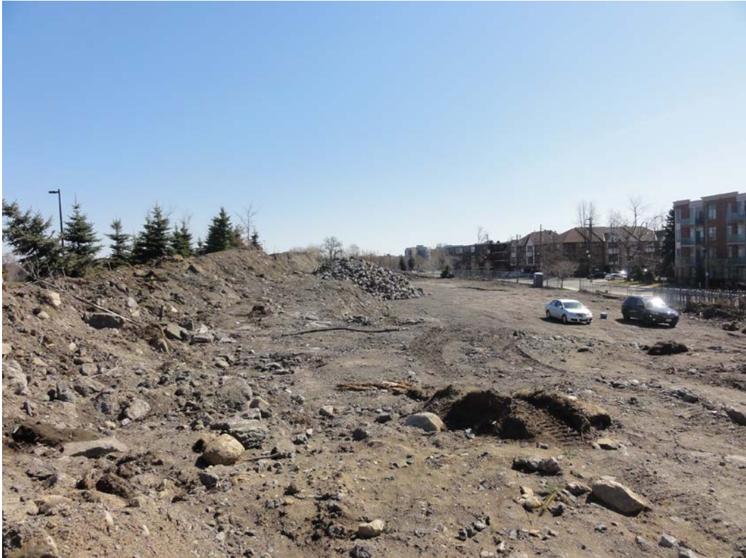
Photo 6: Looking southeast from the northern property line over the Phase One Property (April 22, 2013).
