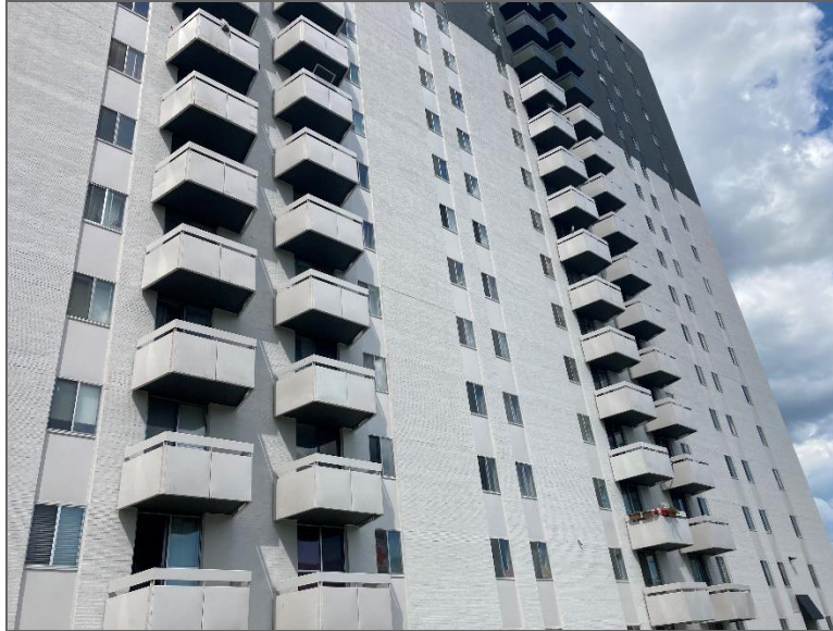
Photo 3 – Site Building B (southeast elevation).
