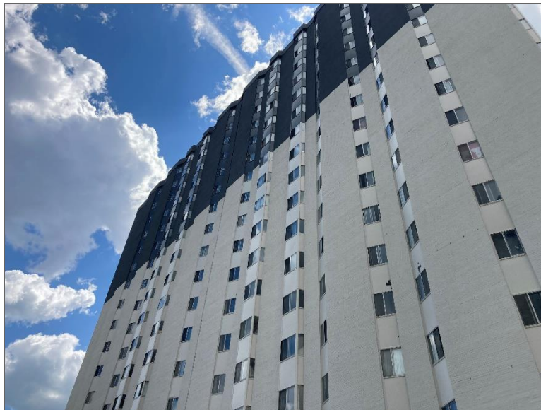
Photo 2 – Site Building A (northeast elevation).
