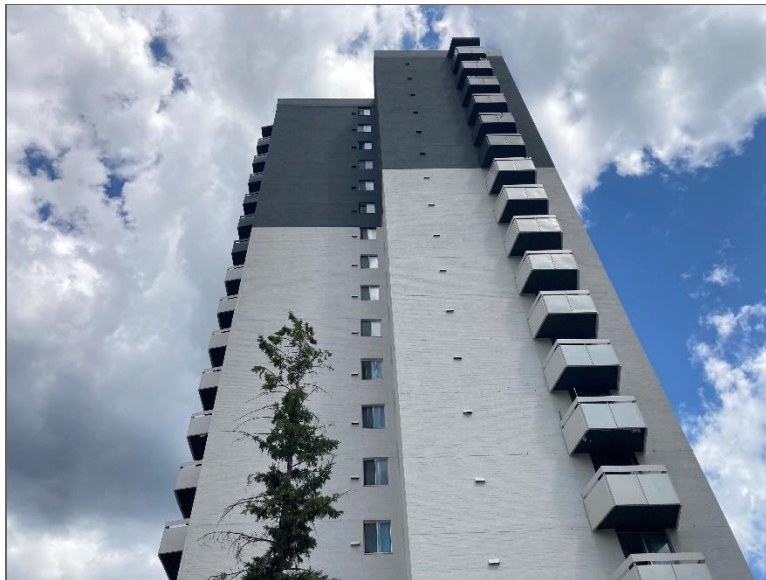
Photo 4 – Site Building B (southwest elevation).
