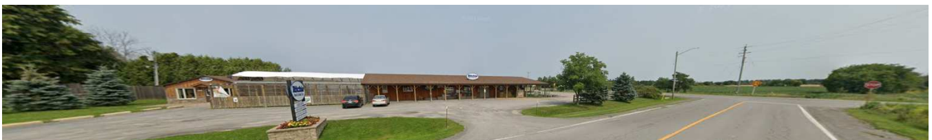
Image 10. Nearby light industrial use looking northeast from Ottawa Street
