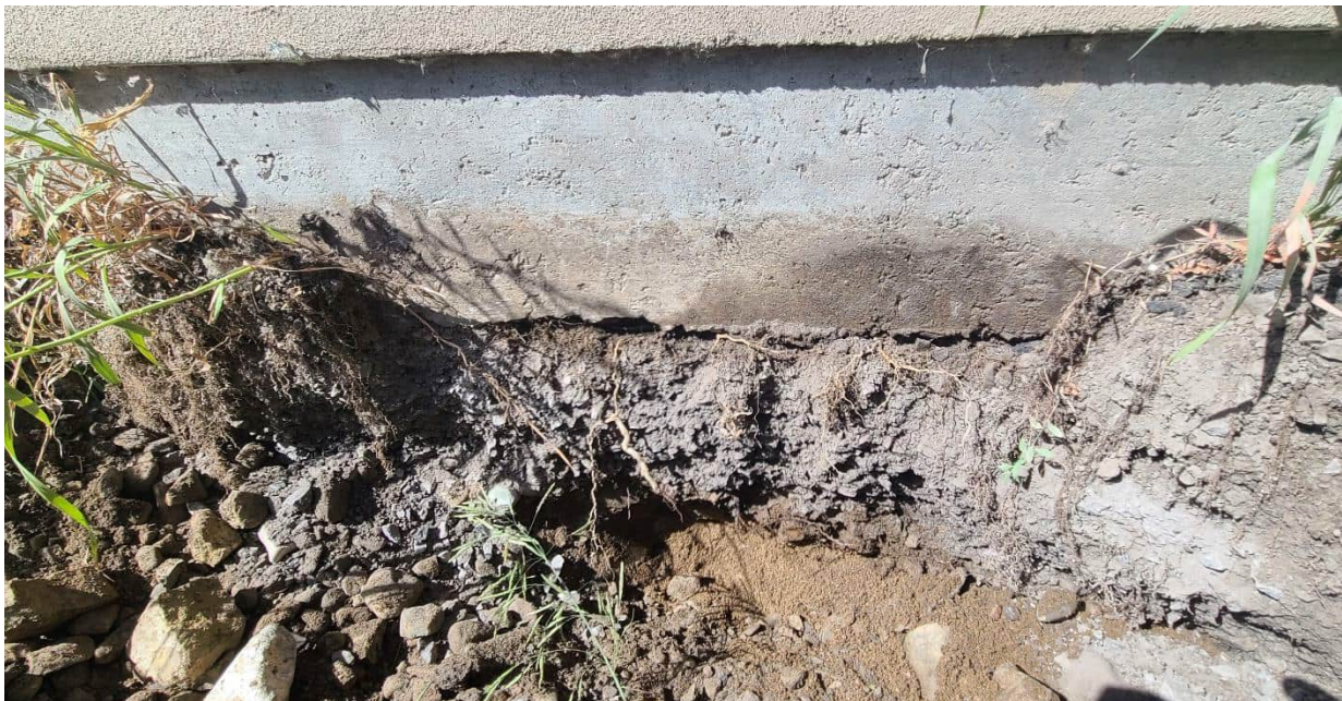
Photograph No. 2: Detailed view of thickened structural slab and subbase materials in Test Pit No. 1
