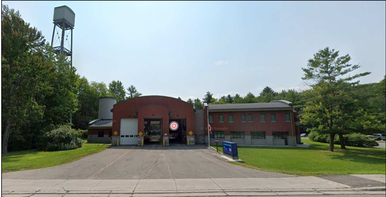
Figure 4. Fire Station and Water Tower along Innes Road
