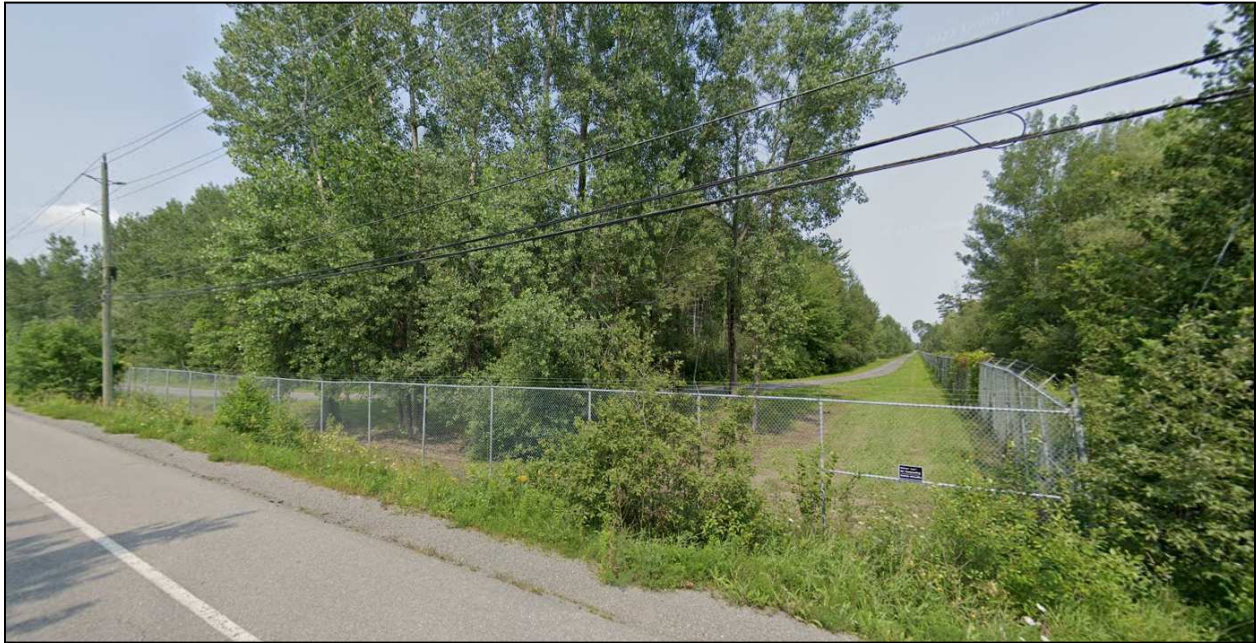
Figure 2. Fenced Federal Lands along Innes Road
