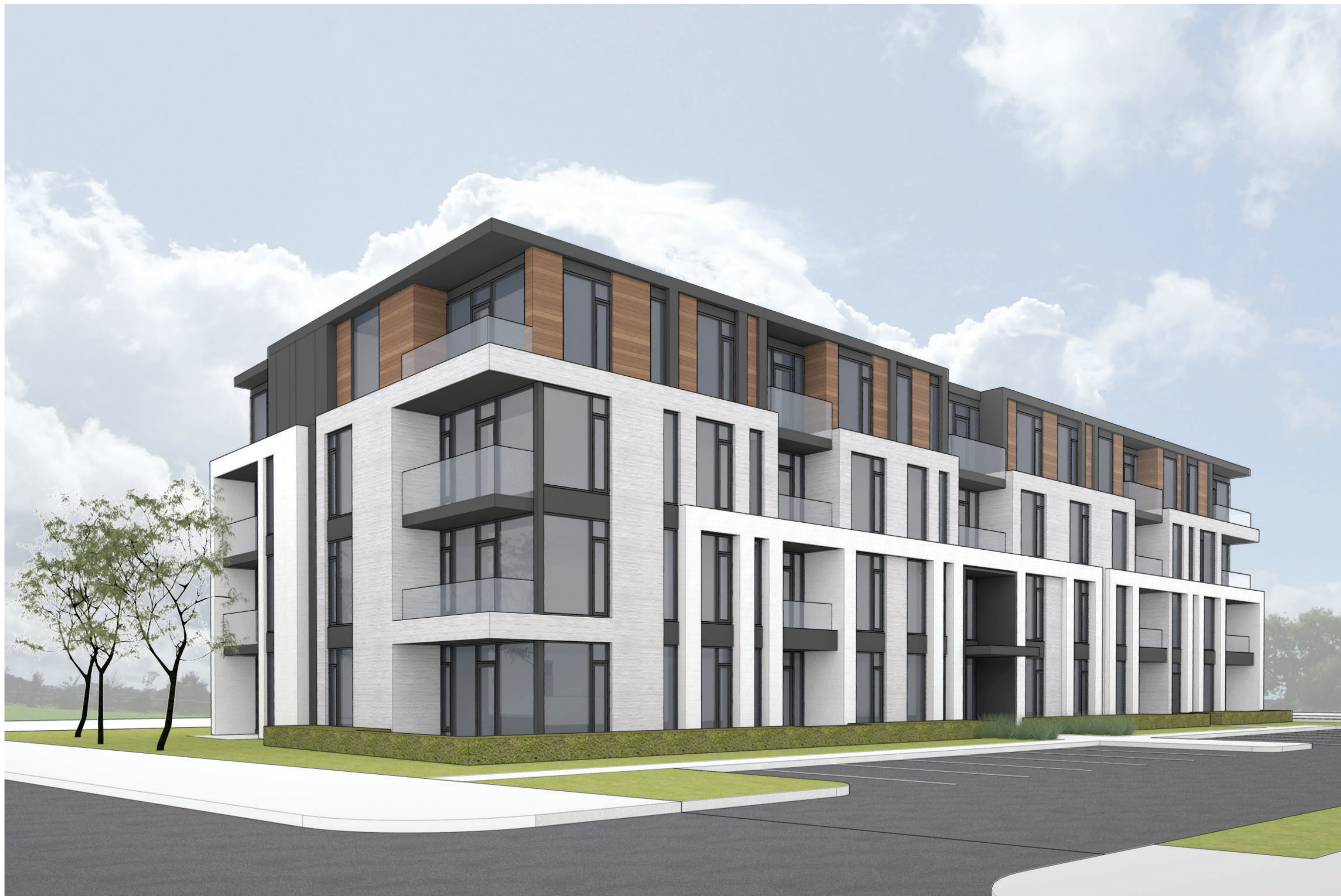
3040 INNES ROAD VIEW OF NORTH-WEST CORNER OF PROPOSED BUILDING
