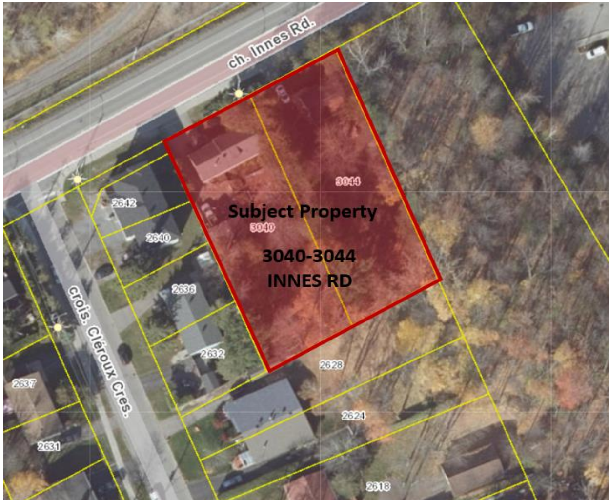
Figure 1: Aerial View of Proposed Development
