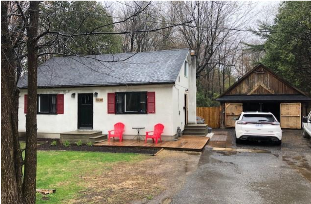
Photograph 1: View of the front of the residential dwelling and storage area addressed 3044 Innes Road on the subject site, facing south.
