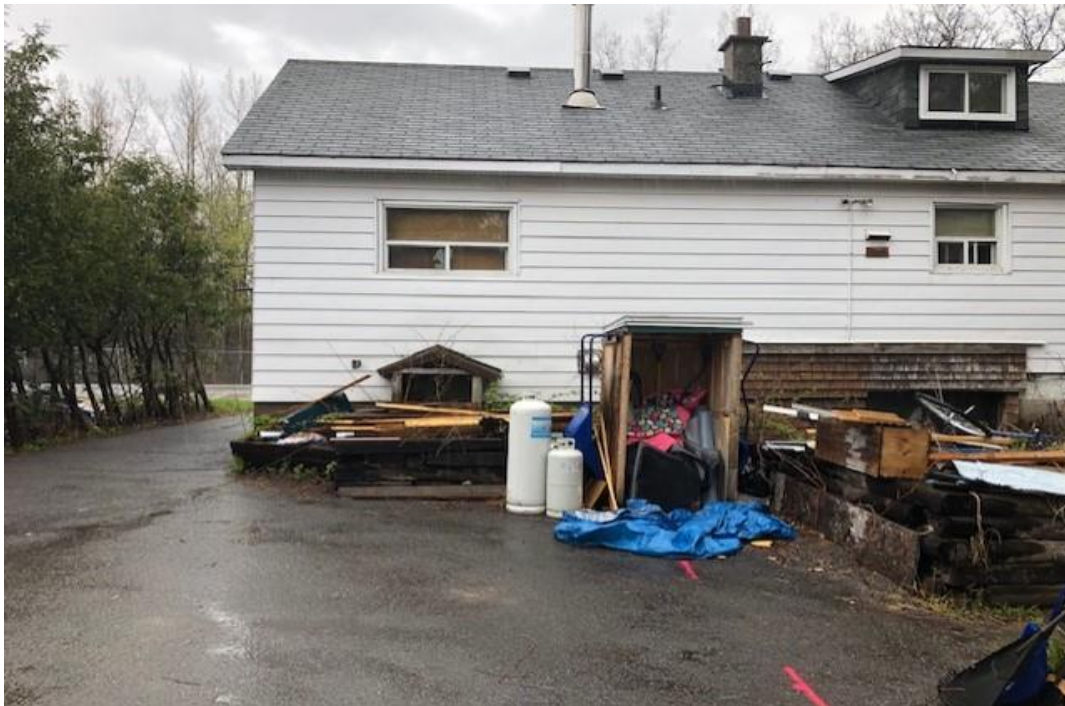
Photograph 2: View of the back of the residential dwelling addressed 3040 Innes Road, facing north.
