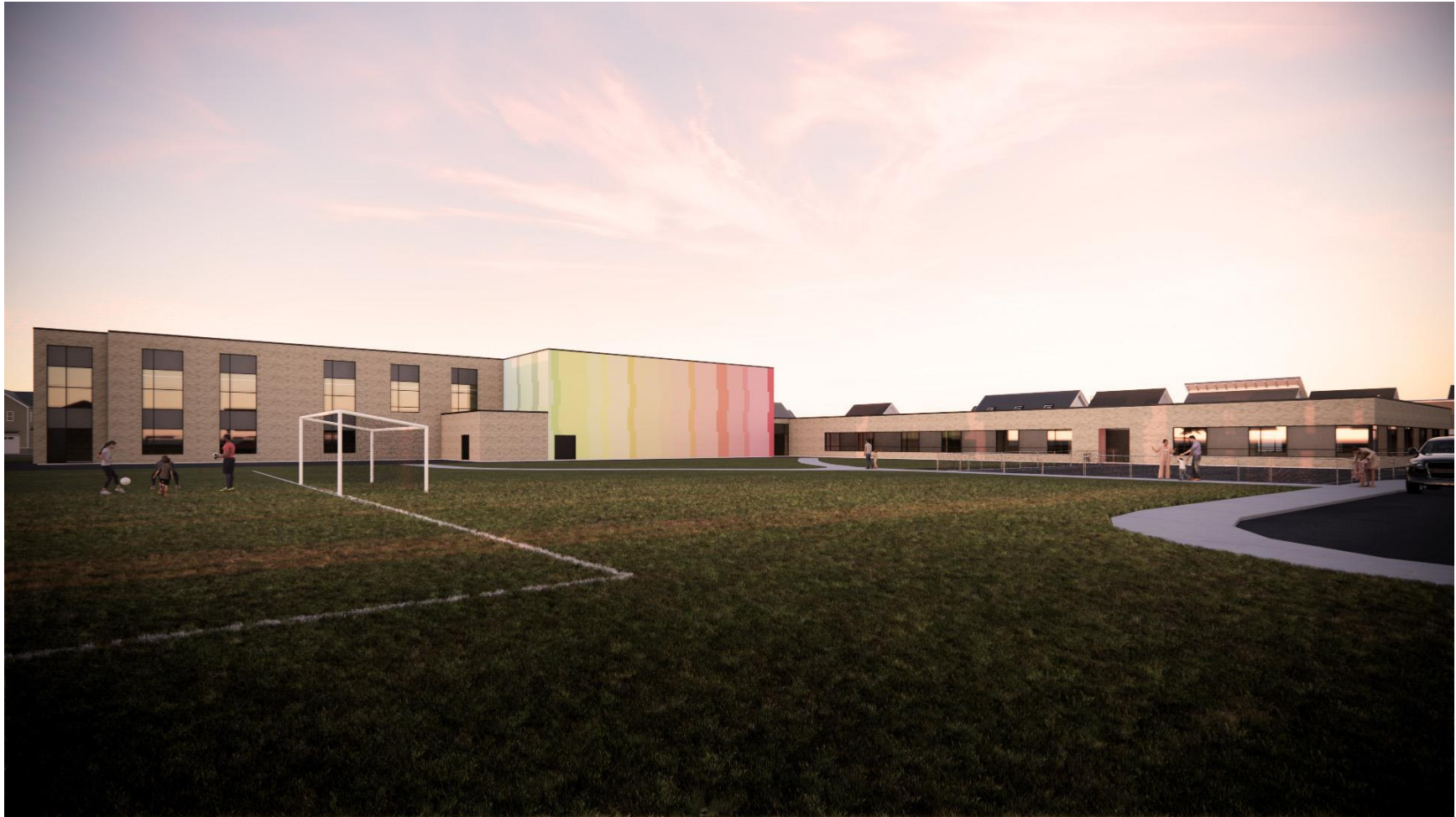
Figure 3-6: Preliminary Rendering – 1045 Kilbirnie Drive – Rear of Building, looking northeast (prepared by Architecture 49, April 2022)
