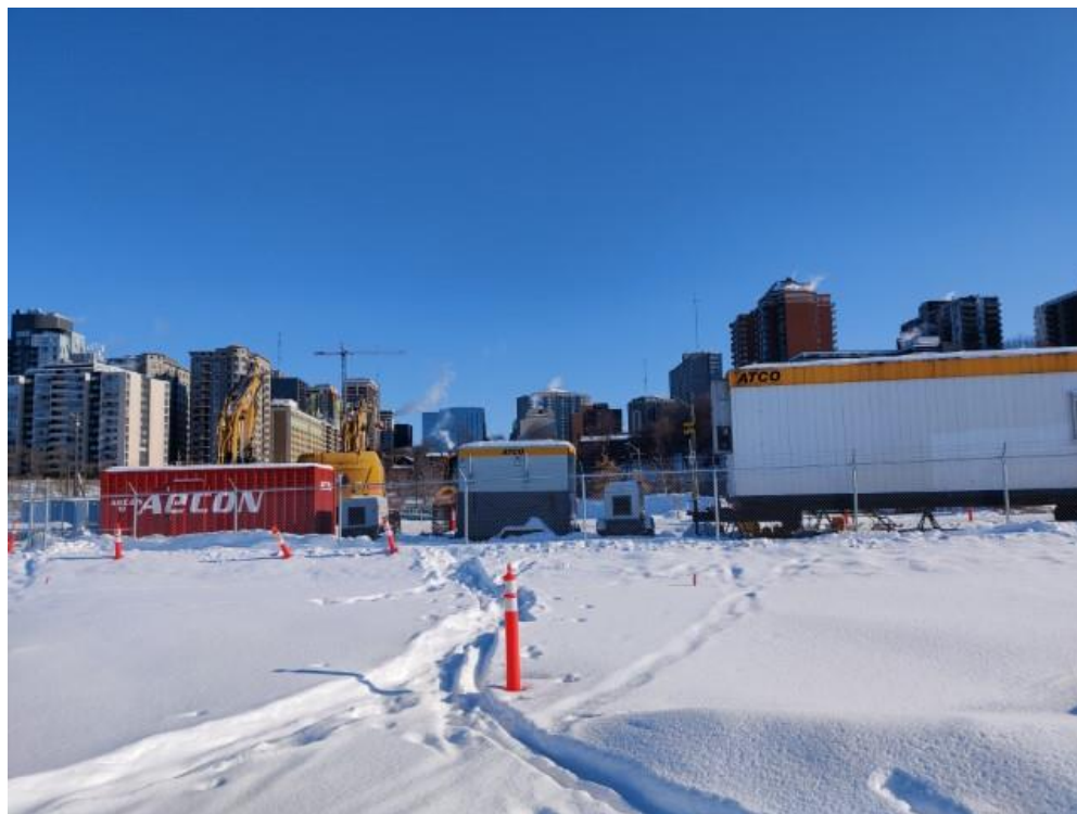
Photo 1: Looking east from eastern side 02
