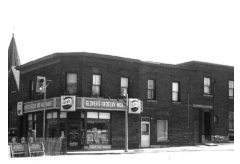
Buildings located on east side of Booth, between Albert and Wellington, 1962. Source: Ottawa Archives
