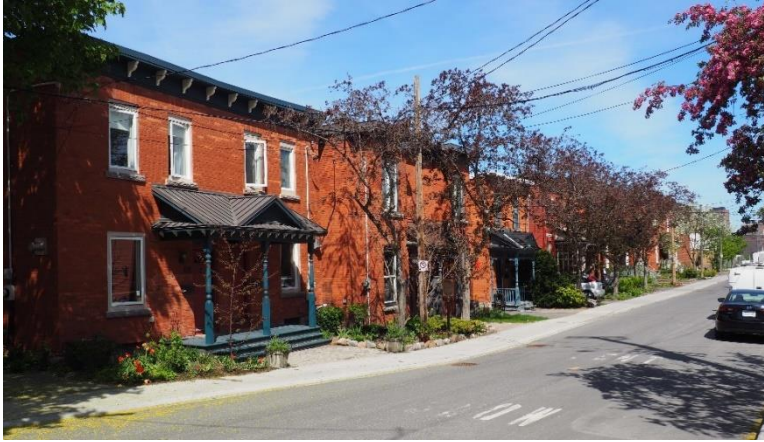
Figure 18: Lorne Avenue (west side), in the Lorne Avenue HCD. Source: Contentworks, 2020.
