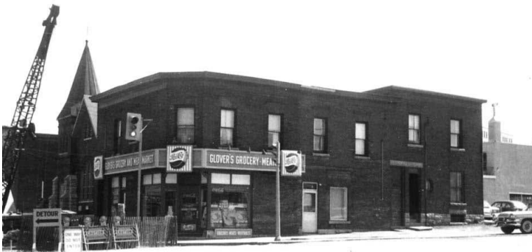
Figure 12: Buildings located on the east side of Booth Street between Albert and Wellington street, on the site what is now 665 Albert Street, in 1962. Source: City of Ottawa Archives, CAO CA 21054, reproduced in Past Recovery Archaeological Services, Stage 1 Archaeological Assessment of LeBreton South, Parts Lots 39 & 40, Concession A, Ottawa Front , 2012: Image 17.
