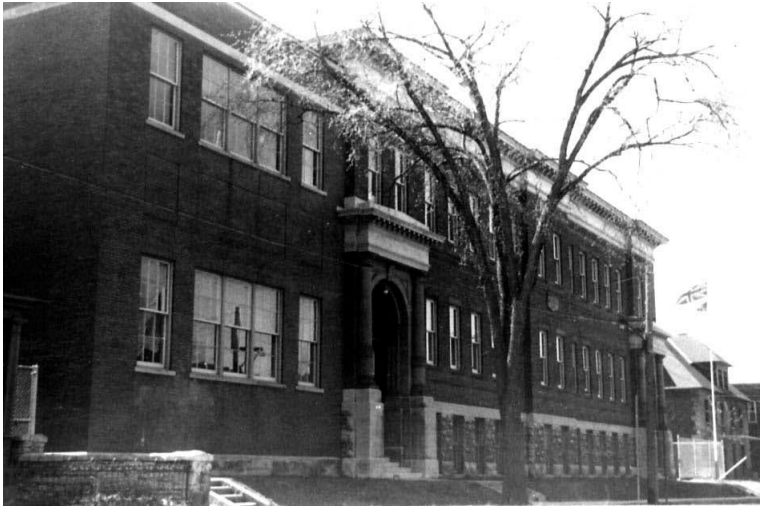
Figure 10: Wellington Street School, built after the fire of 1910, and located on the 665 Albert Street on the site of what had been the Charles Pinhey estate. Photo taken in 1962. Source: City of Ottawa Archives, CAO CA 21047, reproduced in Past Recovery Archaeological Services, Stage 1 Archaeological Assessment of LeBreton South, Parts Lots 39 & 40, Concession A, Ottawa Front , 2012: Image 14.
