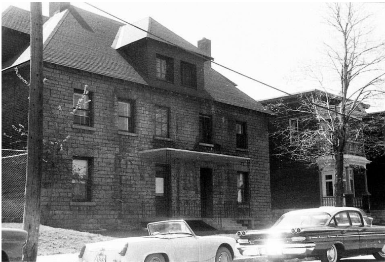
Figure 11: Stone residence located at 646 to 648 Wellington Street, part of the property at 665 Albert Street, 1962. Source: City of Ottawa Archives, CAO CA 21049, reproduced in Past Recovery Archaeological Services, Stage 1 Archaeological Assessment of LeBreton South, Parts Lots 39 & 40, Concession A, Ottawa Front , 2012: Image 15.
