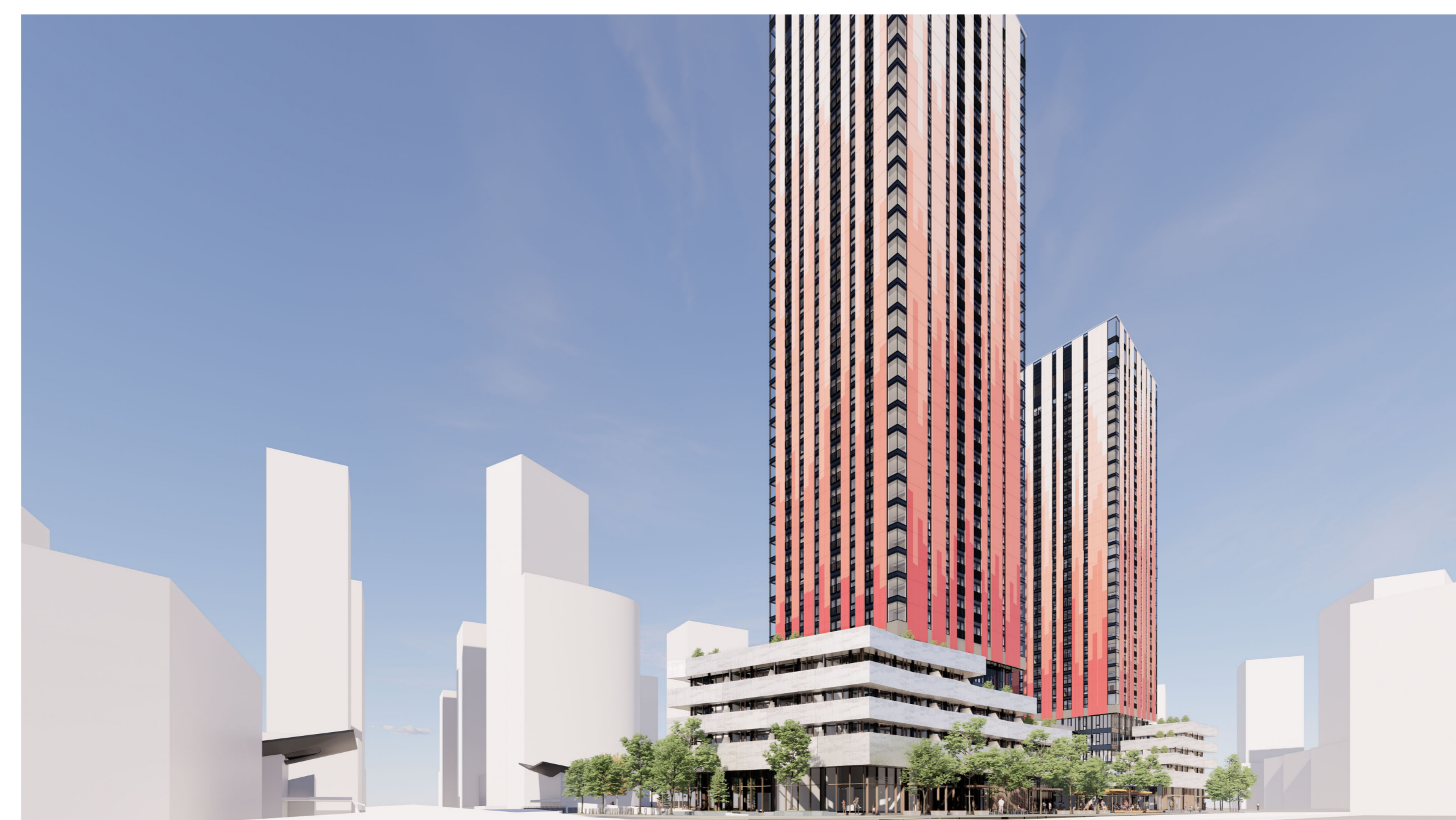
VIEW FROM CORNER OF BOOTH STREET AND ALBERT STREET LOOKING NORTHEAST
