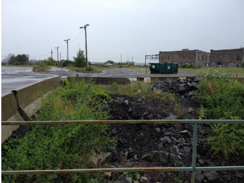
Photograph 11: Fill material observed west of Building #511, facing west (August 12, 2014).
