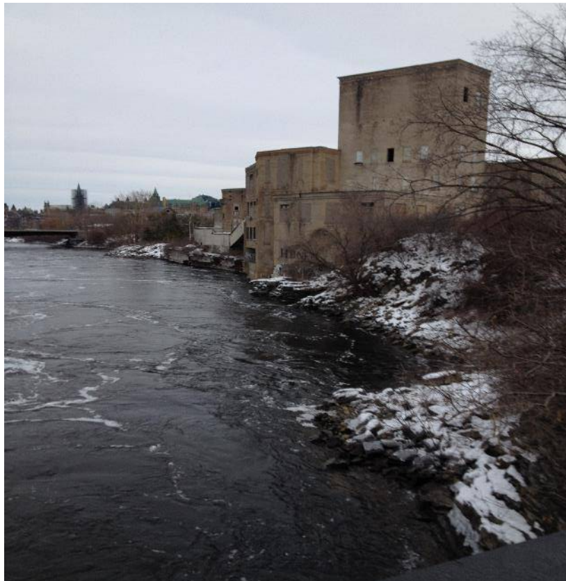
Photograph 4: View of north side of former board mill, facing southeast (April 7, 2014)
