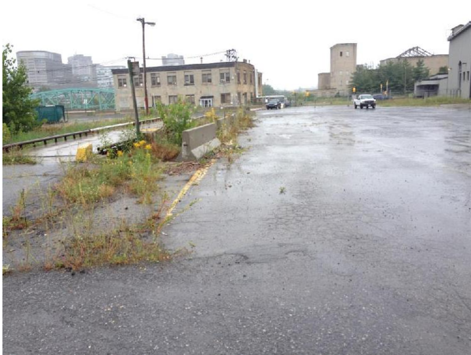
Photograph 12: Paved area with sparse vegetation near northern property boundary, facing east (August 12, 2014).
