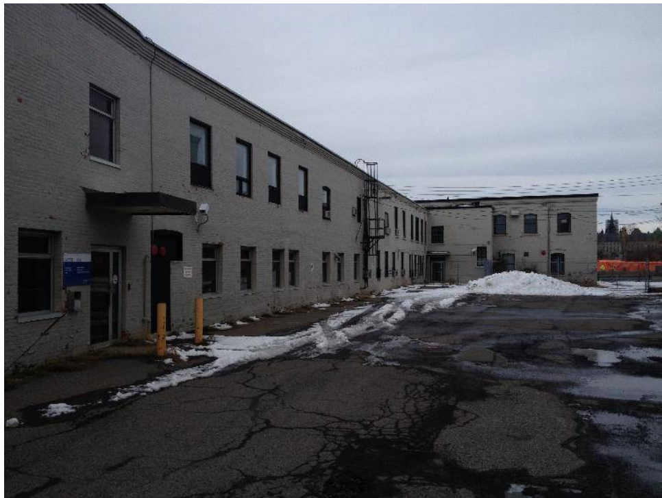
Photograph 2: View of south side of Building 541 and west side of Building 540, facing east (April 7, 2014)
