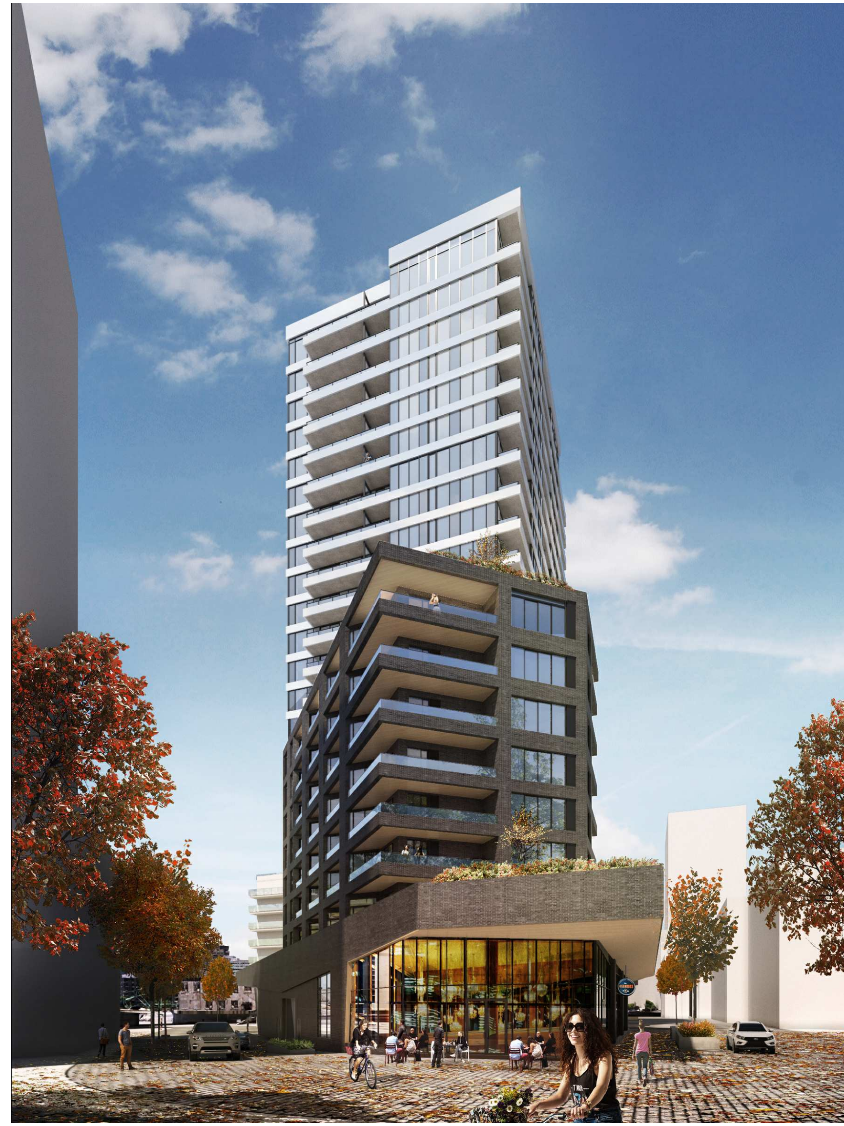
VIEW FROM SOUTH WEST
