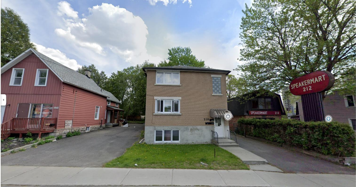
Figure 1: 216 McArthur Ave – Existing Building
